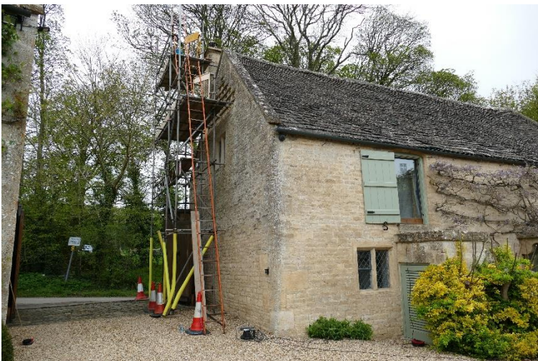
Photograph 1.3 The Stables – Western & Southern Elevations
