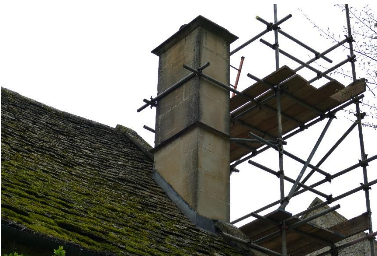
Photograph 1.5 Ashlar stack – Northern and Eastern aspects
