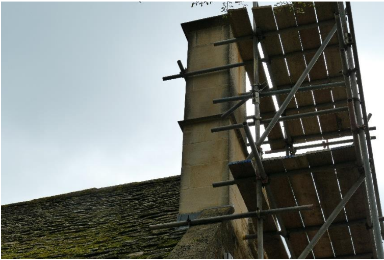
Photograph 1.4 Ashlar stack – Northern aspect
