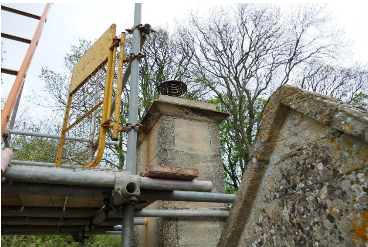
Photograph 1.6 Ashlar stack – Southern aspect
