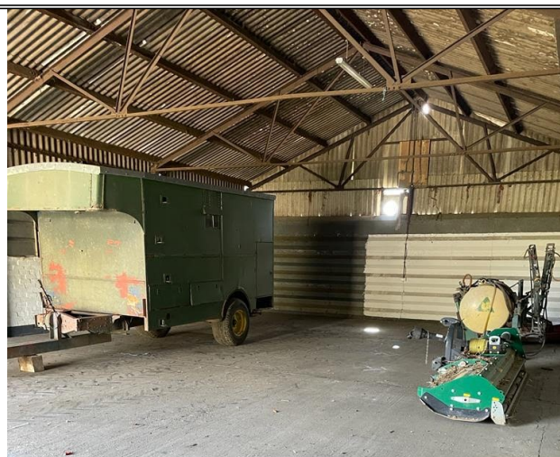
Image 2: Interior of Existing Agricultural Shed, Storing Agricultural Machinery
