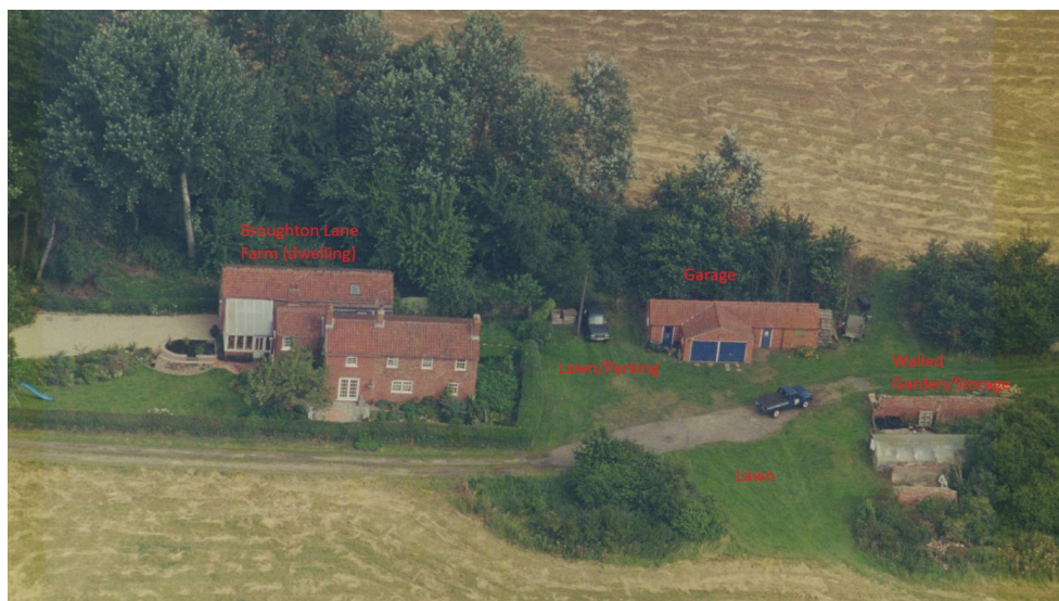
Aerial photograph dated 1999 depicting use of application site to east of dwelling as lawn, car parking area, ancillary garage and walled garden/storage.
