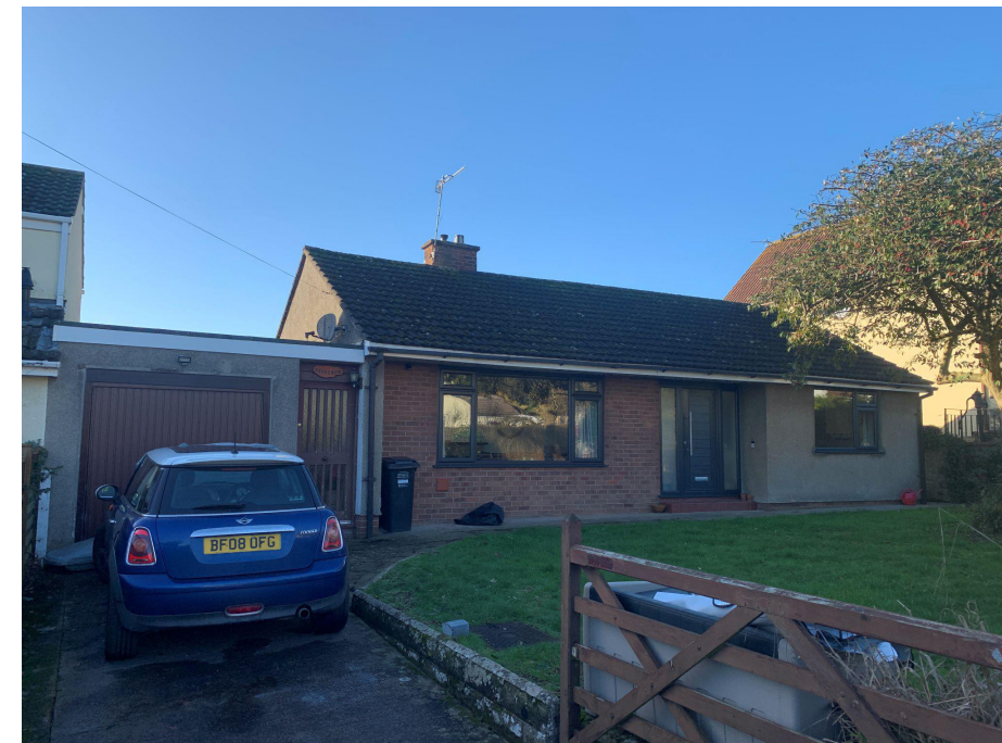
Photograph of the front of the property
