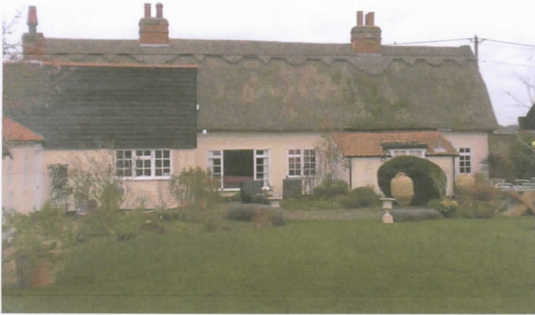
Partial view of rear elevation, showing black weatherboarded kitchen area where proposed new extension will abut up to, and will be re-clad with new horizontal timber cladding. Oblique view of existing 'rear wing' which is proposed to be extended.
