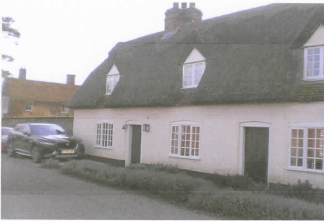
Partial view of front elevation (unaffected by proposed works)
