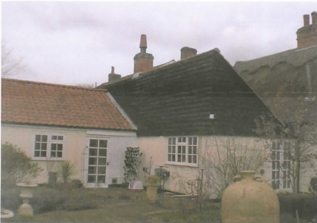
Partial view of 'rear wing' and existing kitchen area (extension proposed to front / to join kitchen area, with this to receive new window and replacement timber cladding above ground floor window head level)
