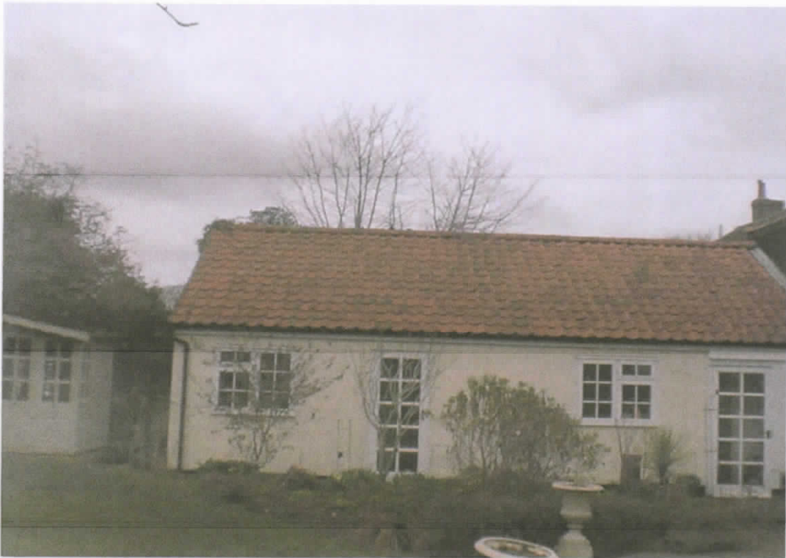
Partial view of 'rear wing' existing (extension proposed to front)
