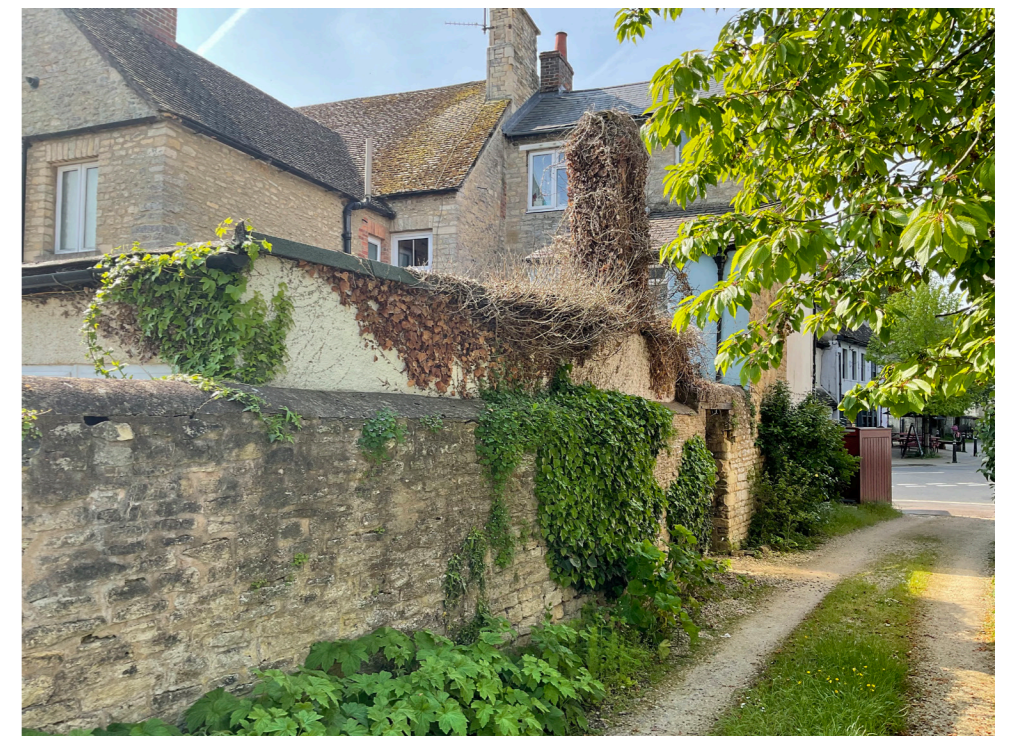
Single storey building at rear (garden building)
