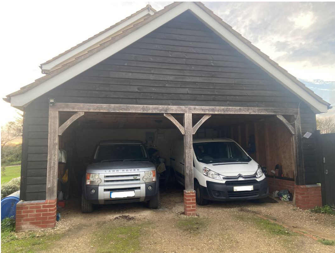
Side Elevation showing existing 2-bay garage – full length windows are proposed to one bay and a door and a small window to the other
