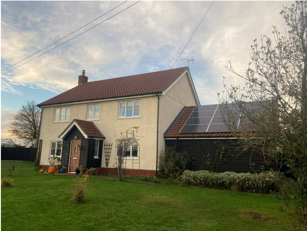
Front Elevation showing existing attached garage to the side – one window is proposed to the front elevation which will match the existing windows on the house
