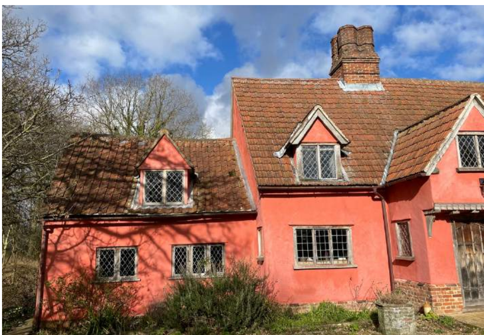
Figure 3 – Barfords from the front- the smaller single cell annexe to the west on the left
