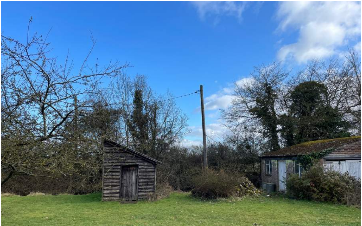
Figure 6 – Barfords timber outbuilding to the rear.
