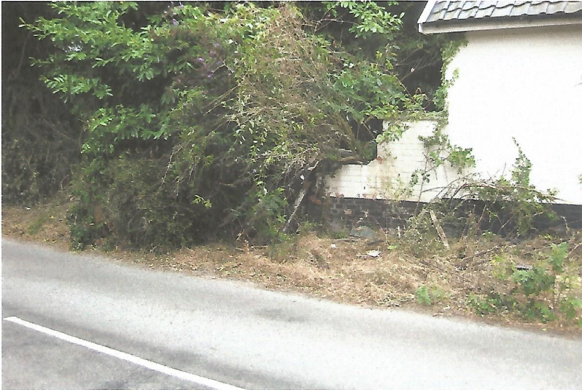
Picture 1 Damage to brickwall and lychgate looking from road
