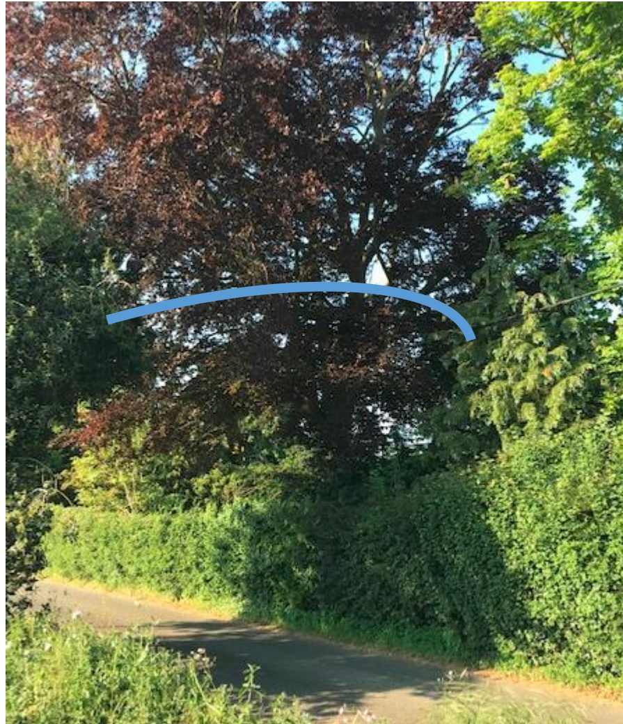
Photo A: Shows tree overhanging road and tangled with electrical supply
