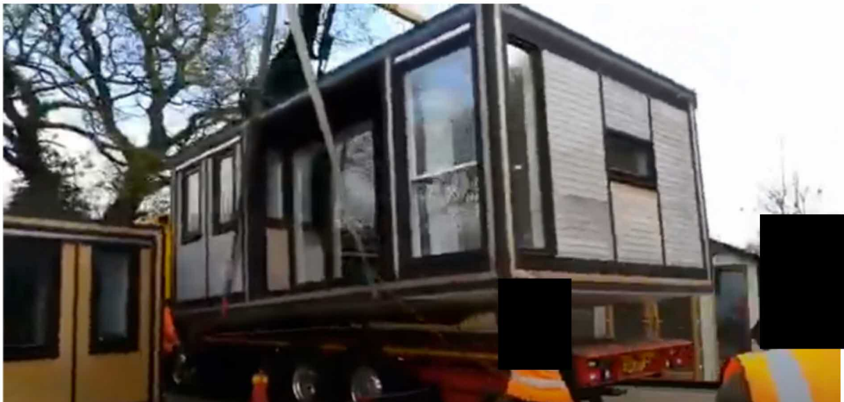
Figure 1 Removal of annexe by truck/hoist
