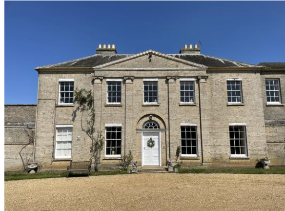
Front elevation of The Old Rectory
