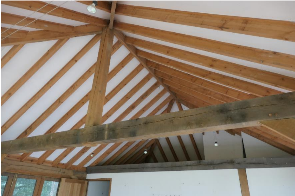
Photo 9 , internal view of building one, looking west.
