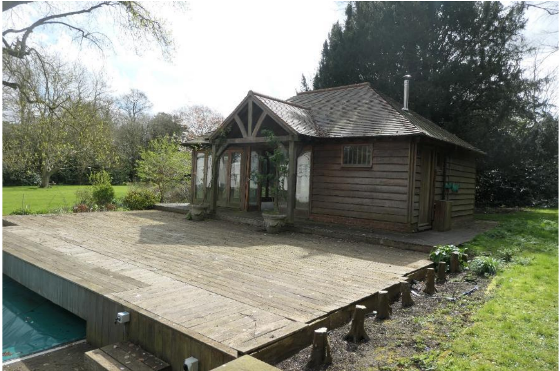
Photo 5 , building one and hardstanding within survey area D, looking southeast.
