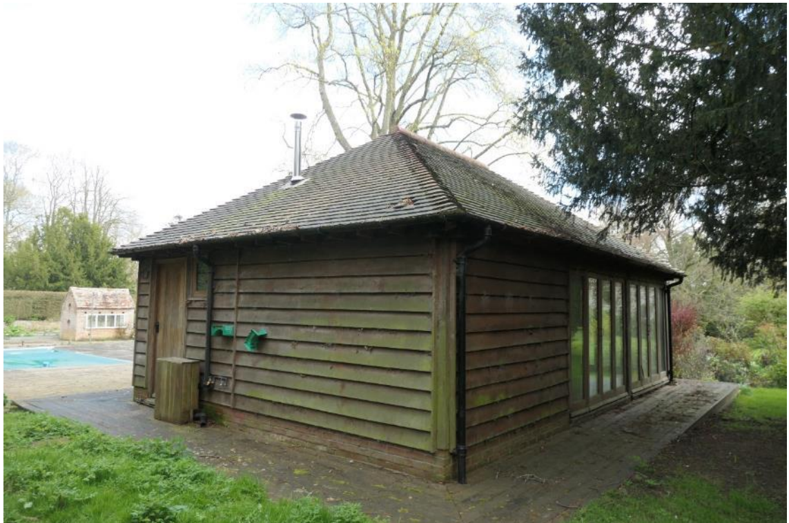
Photo 8 , south and east aspect of building one located within survey area D, looking northeast.
