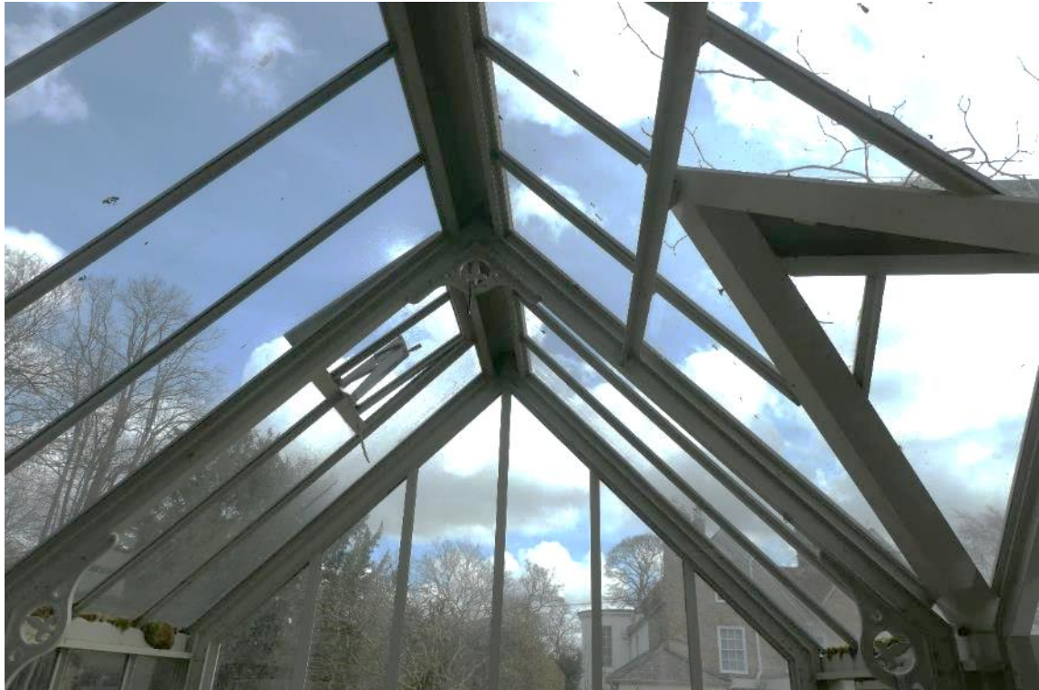
Photo 12 , internal view of building two, looking east.
