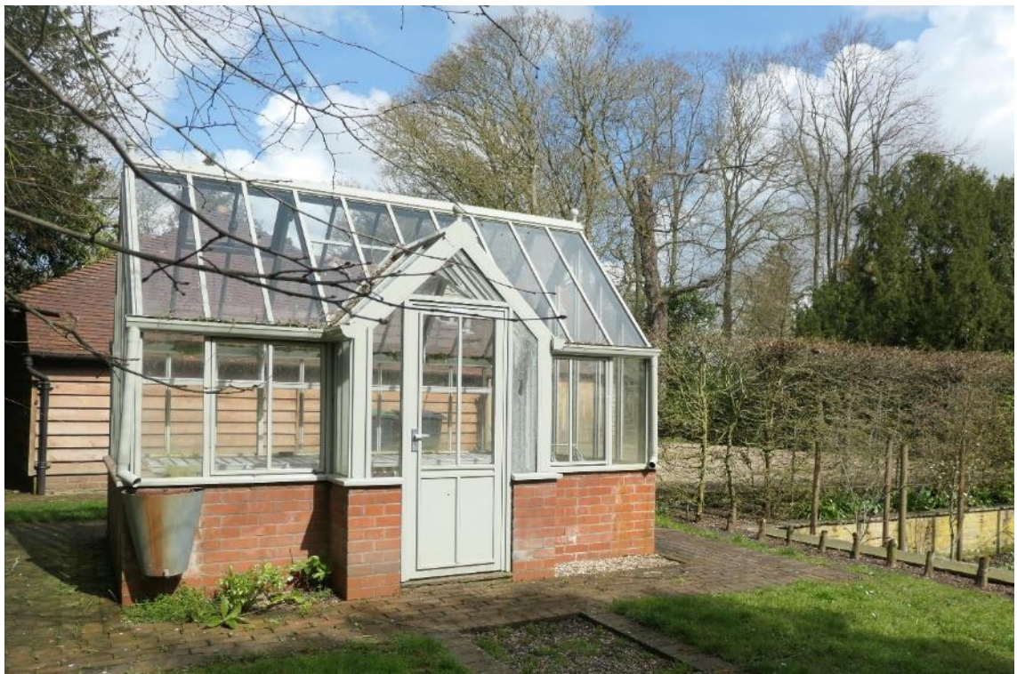
Photo 6 , hardstanding and building two within survey area C, looking north.
