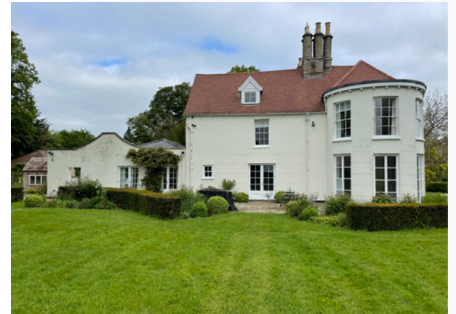
View of wall in context of south elevation
