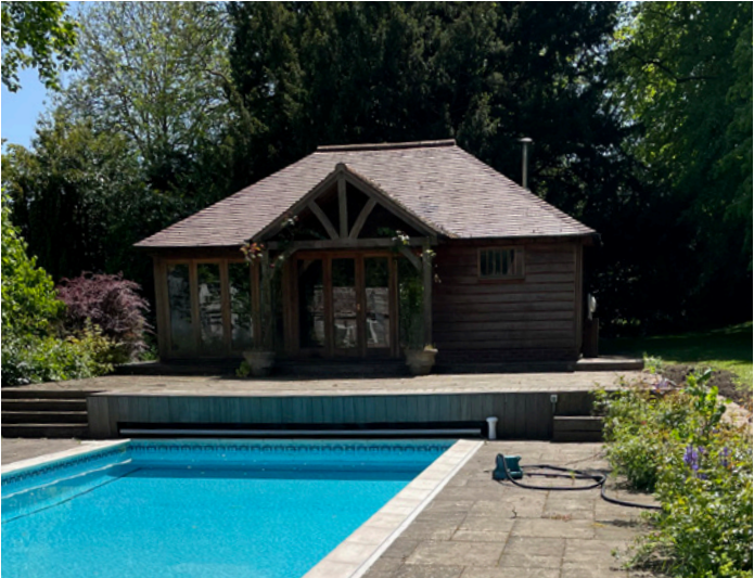
View of the existing Pool House building for demolition/removal
