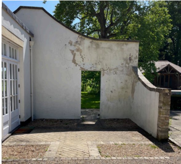
View of wall abutting kitchen for removal
