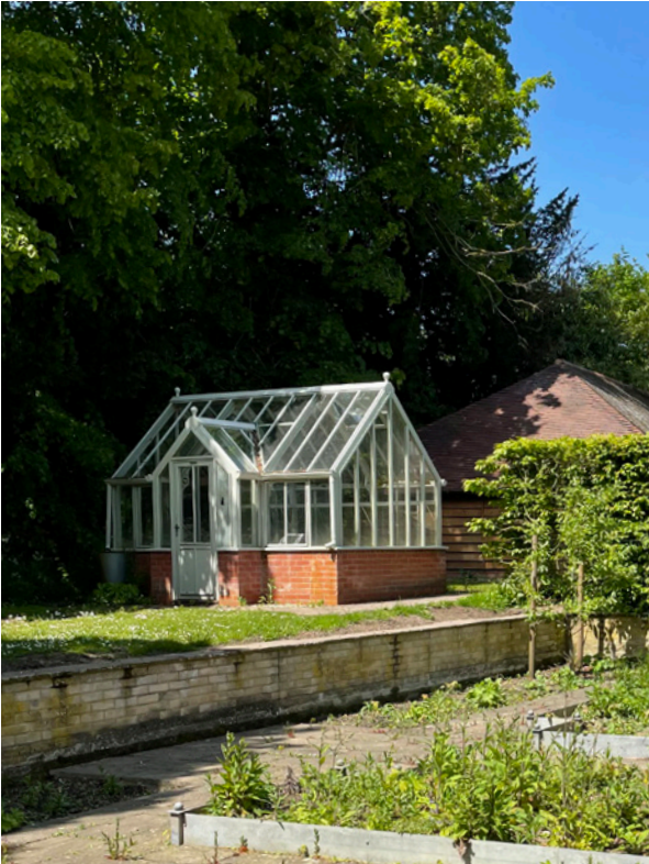
View of existing aluminium Greenhouse for demolition/removal/
