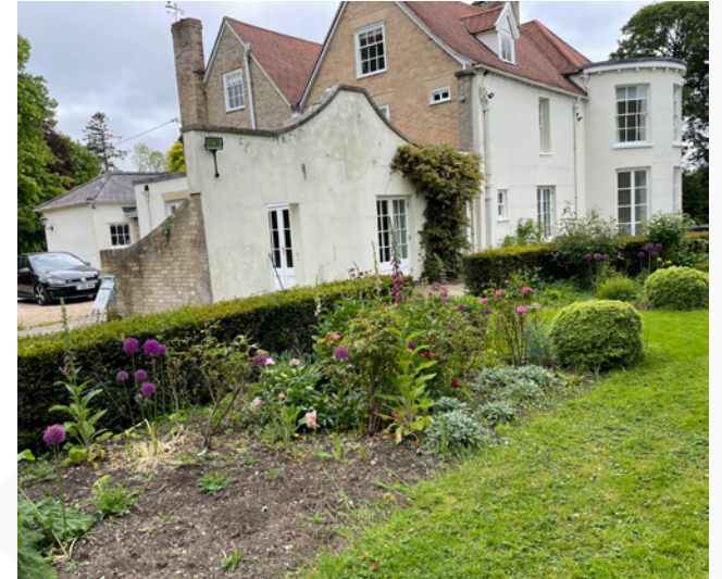
View of wall abutting kitchen for removal looking north
