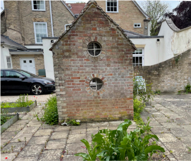
View of the west elevation
