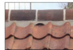
Gap beneath raised clay ridge tile
