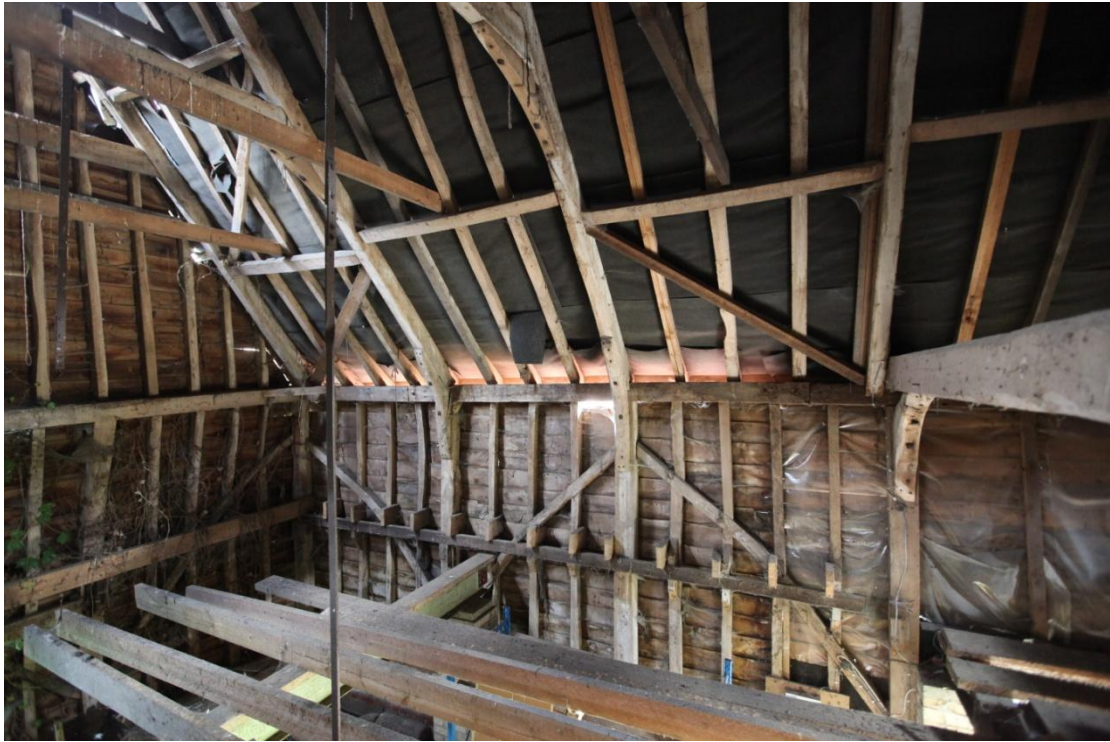
Figure 25. The eastern interior of the barn's three narrow northern bays (1) showing the staggered butt-purlins of the roof structure and the intact wall studs interrupted by curved diagonal braces.
