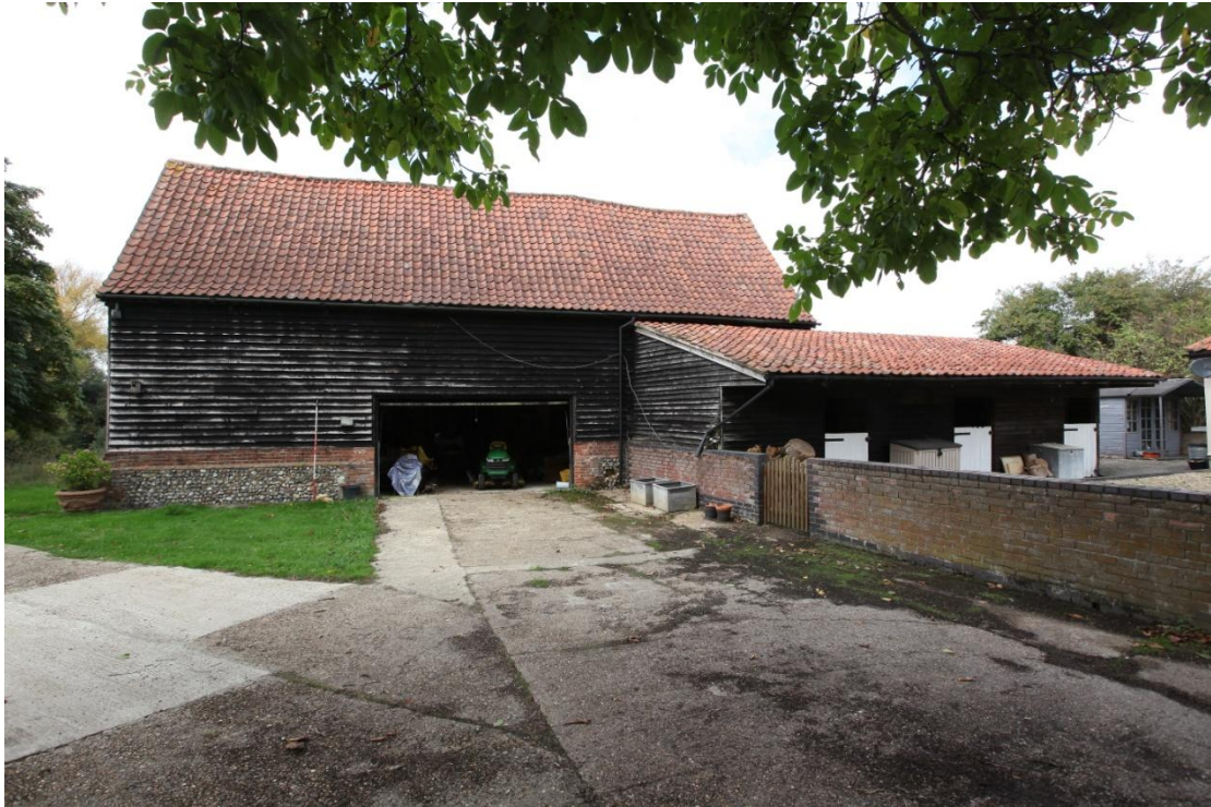
Illus. 5. The barn (1) from the east showing the pantiles that are likely to have replaced thatch and the tarred weatherboarding on a plinth of flint-rubble and brick. The present ‘up-and-over’ garage-type door occupies the position of the original full-height central entrance but extends further to the left. The lean-to former stable (2) on the right consists of modern softwood and dates only from the late-20 th century, having replaced a smaller open-fronted shelter-shed shown on 19 th century maps.
