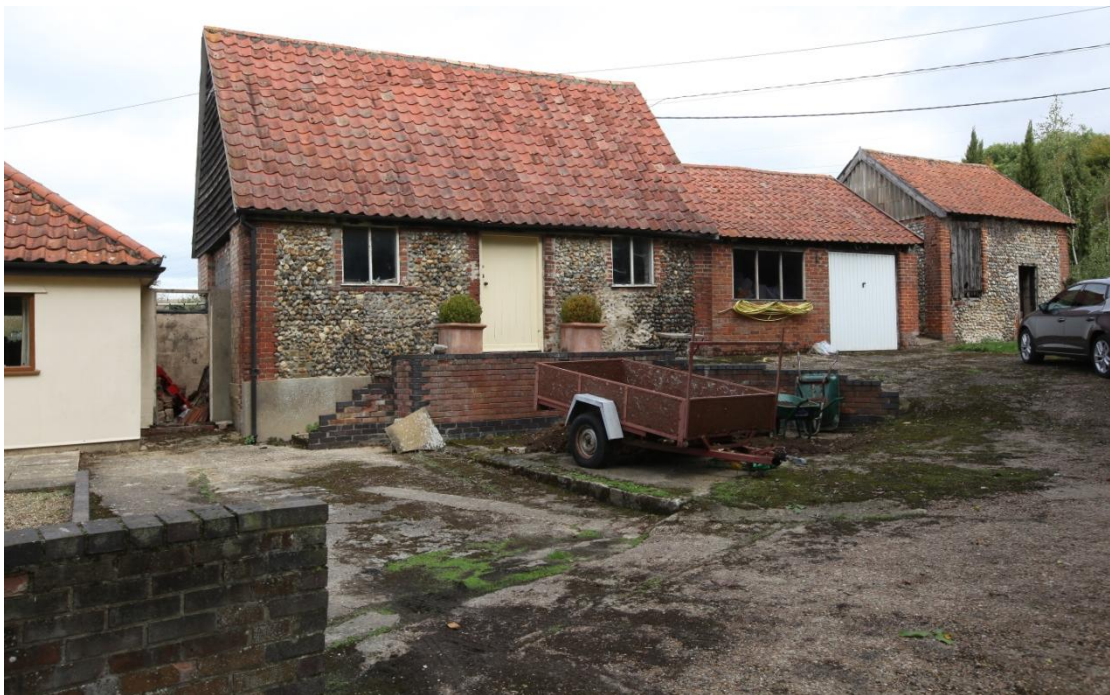
Illus. 4. The southern facades of the farm buildings to the east of the linear range, with the central entrance and flanking windows of the early-19 th century flint-rubble apparent stable on the left (5). Its steeply pitched roof suggests it was initially thatched. The low central shed (6) has been largely rebuilt in 20 th century brickwork to form a garage but the detached 19 th century flint-rubble shed to the right is an unusual building originally lined with internal vertical boarding that may have formed a tack room with the hatch of an integral chaff box to the left of its entrance. (Included for site context.)
