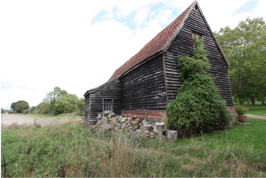
Illus. 7. The barn (1) from the south-west showing the 20 th century window in the southern gable and the original central lean-to rear porch facing the meadow to the west. The steep pitch of the roof indicates it was designed for thatch.
