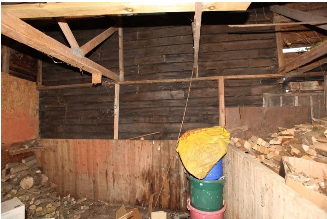
Illus. 10. The ostensibly original tarred elm external weatherboarded to the eastern exterior of the barn's northern bays, protected within the 20 th century lean-to stable (2). The modern softwood rafters and studs of the latter are visible in the foreground.
