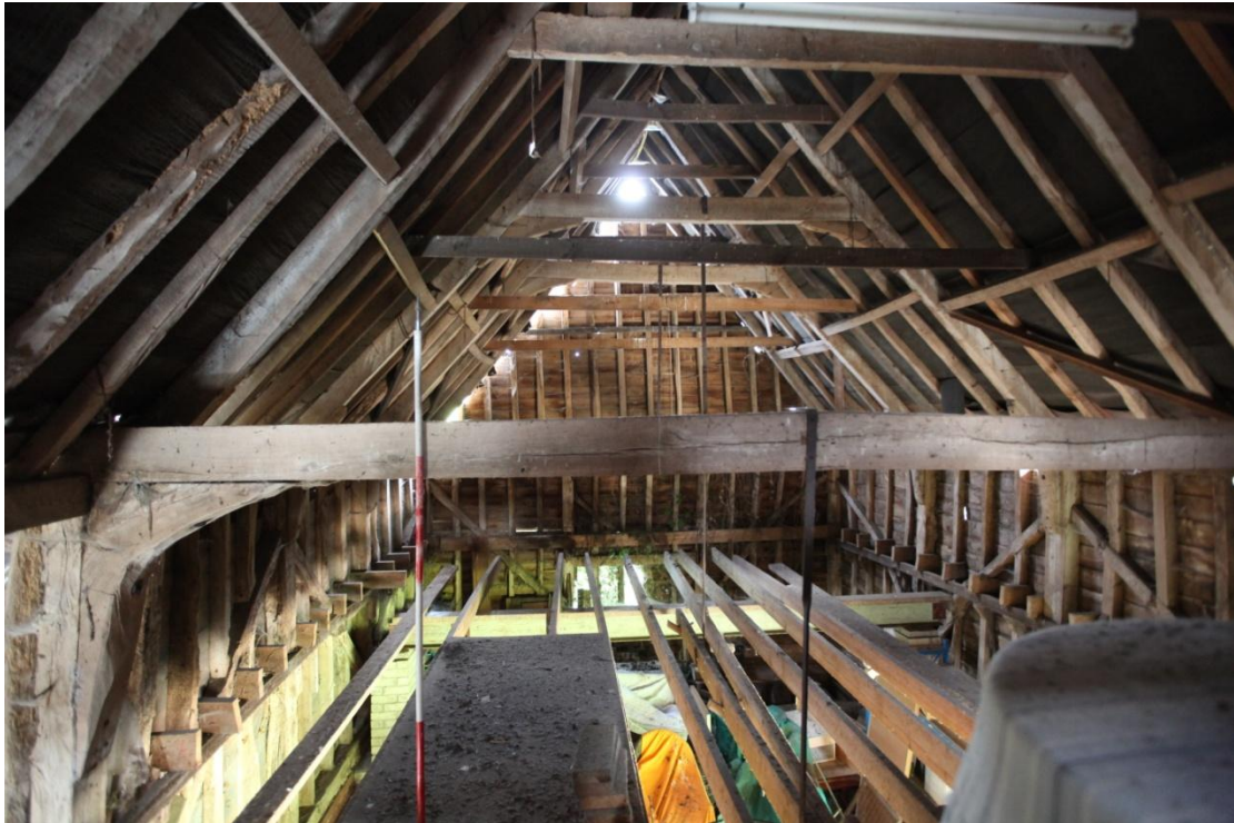
Illus. 23. The northern bays of the barn (1) with the original knee-braced tie-beam defining the central threshing bay in the foreground.
