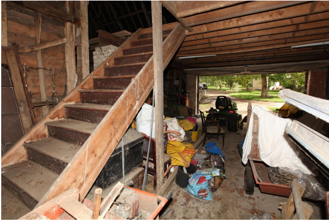
Illus. 19. The rear porch from the west (1), showing the garage-style entrance in the rear and the late-20 th century domestic staircase serving the contemporary loft.
