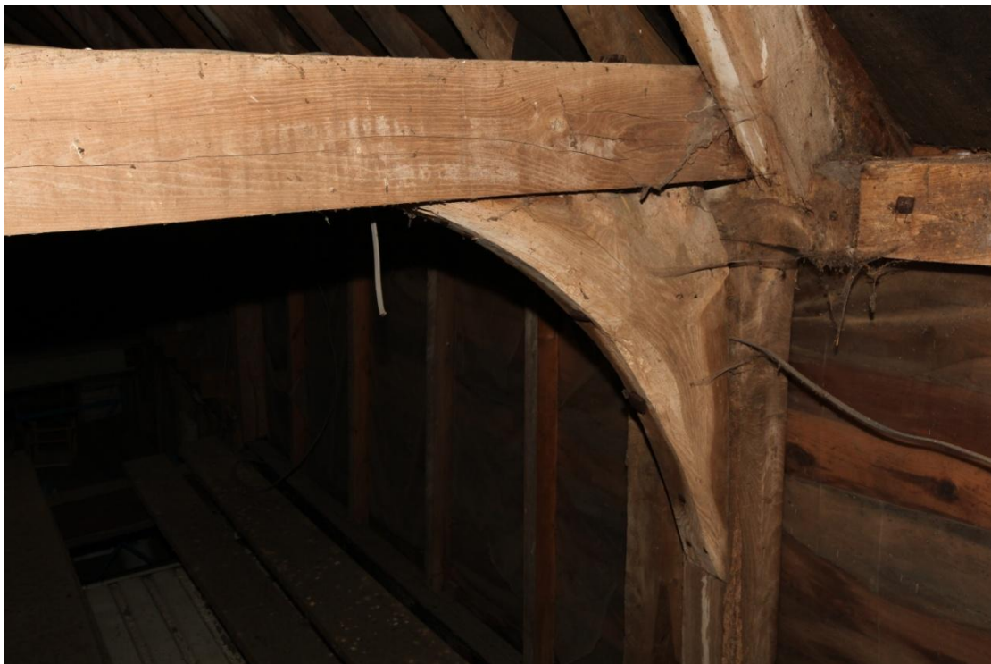
Illus. 36. A detail of the original bolted knee-brace to the south-eastern storey post of the threshing bay showing the distinctive colour and grain of the elm tie-beam with a face-halved and bladed scarf joint in the roof-plate to the right.
