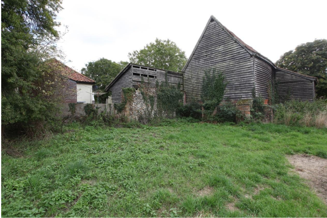
Illus. 9. The 20 th century weatherboarding of the barn's northern gable (1) showing the 20 th century brick buttresses added to the original flint-rubble plinth. The modern lean-to stable (2) adjoining to the left incorporates the flint-rubble western wall of the shelter-shed shown on the historic Ordnance Surveys but structure 3 in figure 9 to the extreme left has been demolished and replaced by a modern cement-block wall and a small boarded shed. The hipped roof of the modern bungalow is visible beyond.
