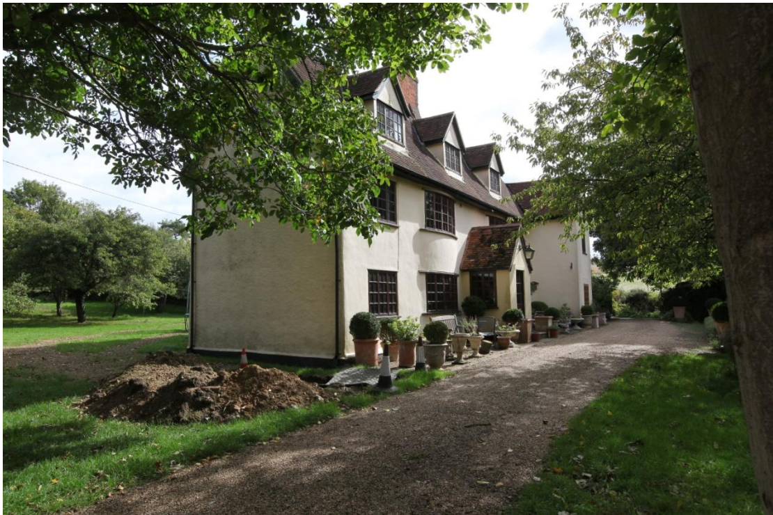
Illus. 2. The former farmhouse from the north-west (included for site context). This timber-framed and rendered three-cell building dates from the early-17 th century but was heavily altered and extended in the late-20 th century and is not listed.
