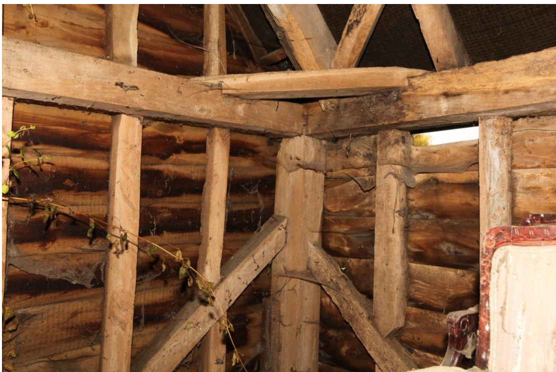
Illus. 32. A detail of the barn's south-western corner to the right in illustration 31 (1) showing the lack of jowl (swollen top) to the post and the tenoned and pegged junction of the gable tie on the left and the roof-plate to the right. The diagonal tie is original.
