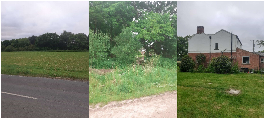
Left: Eastern elevation viewed from Dauby Lane, Centre: Northern elevation viewed from the farm track, Right: Eastern elevation viewed from the garden showing lack of original features
