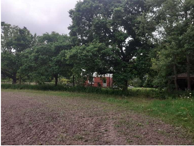
Above: Southern elevation showing eastern side obscured by trees when viewed from the countryside.
