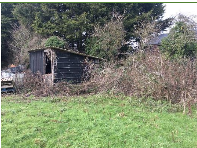
Photograph 5. Scrub on northern site boundary around dilapidated shed.
