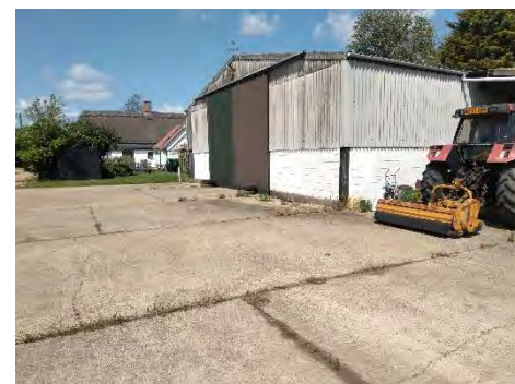
Photo 4 – Overview of the large barn on the site looking north west.
