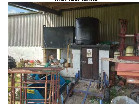
Photo 7 – Overview of the storage area on site with fuel tanks
