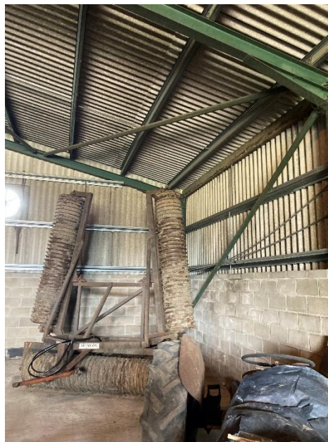
Fig 6 – Internal View of braced portal frame rafters & columns.
