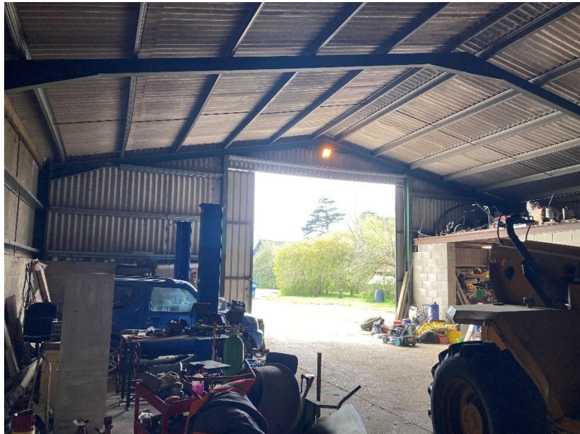
Fig 8 – Internal view of ground bearing concrete floor slab.
