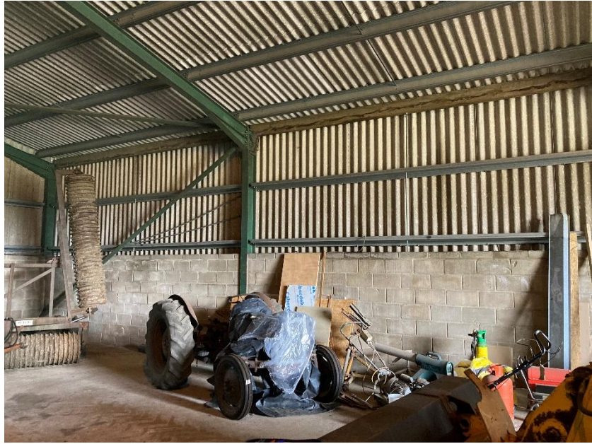
Fig 7 – Internal view of portal frame column & masonry plinth.
