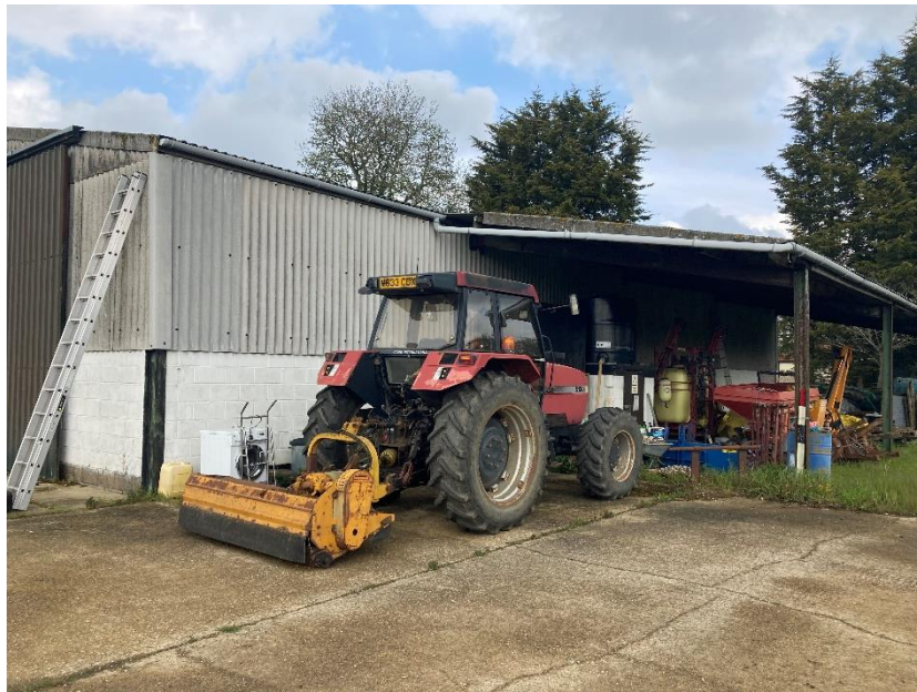
Fig 3 –East Elevation – Side elevation of existing barn, viewed from rear eastern boundary.
