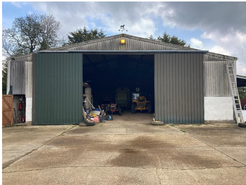
Fig 2 – South Elevation – Front elevation of existing barn, viewed from entrance hardstanding.
