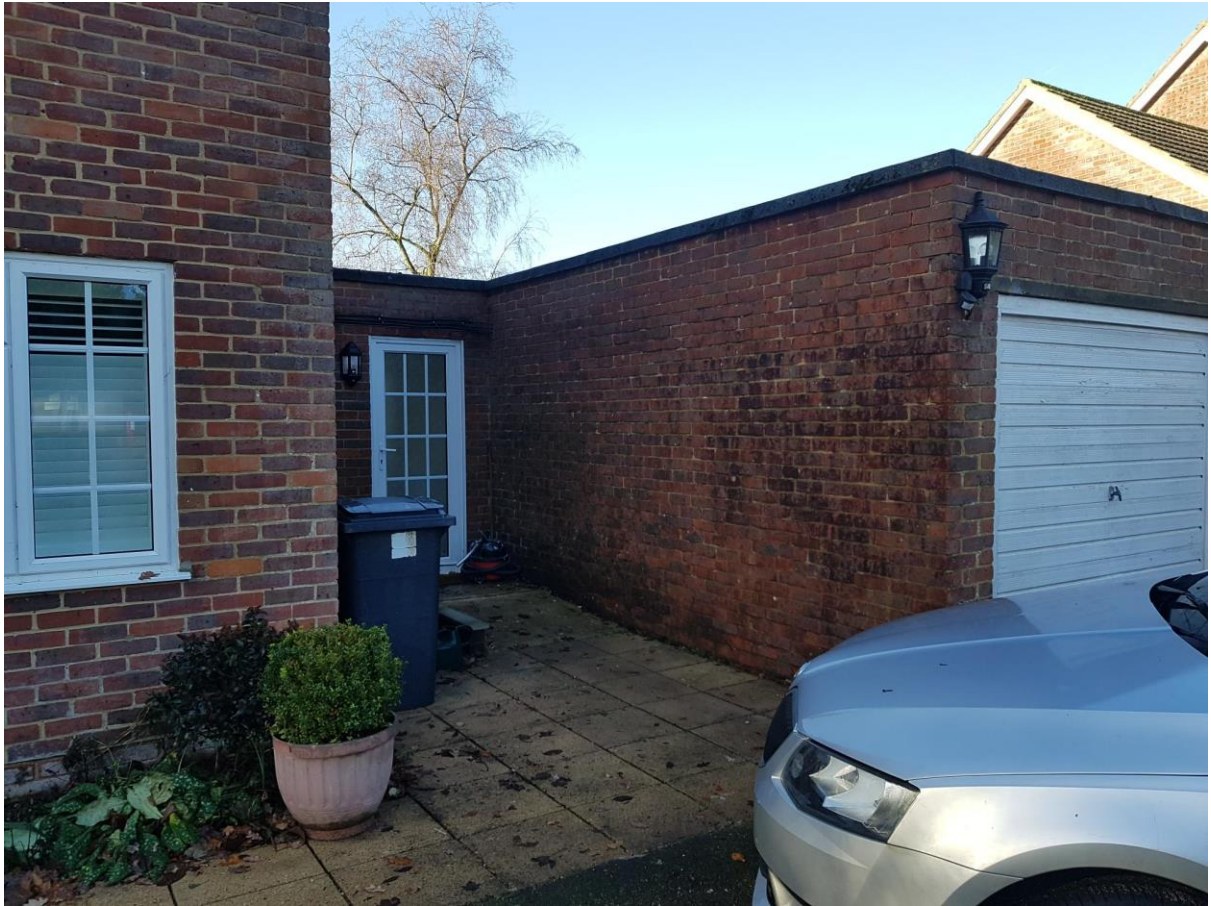
Front Elevation Approach to Utility Room
