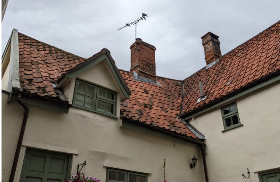
Picture 1: Roof on front elevation
