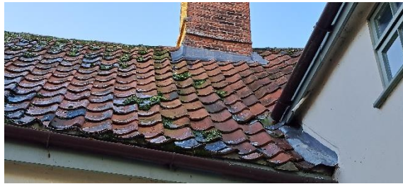
Photo 6 North elevation – raised tiles (scattered ad flashing along junction in roof)
