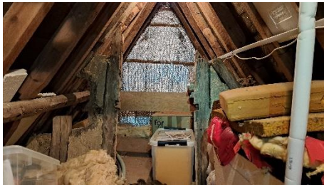
Photo 9 Interior of loft – good condition mortar on brick work on chimney
