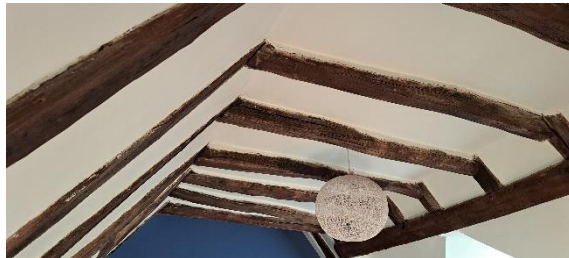
Photo 10 Interior of rooms in north-south section with plastered ceiling and timber beams
