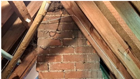
Photo 9 Interior of loft – good condition mortar on brick work on chimney
