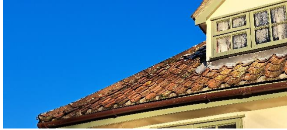
Photo 4 South east elevation showing raised tiles and flashing around chimney
