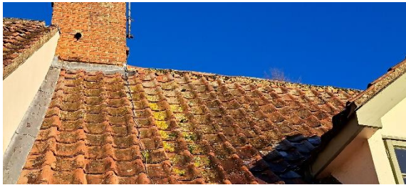
Photo 5 South east elevation – raised tiles and flashing around dormers
