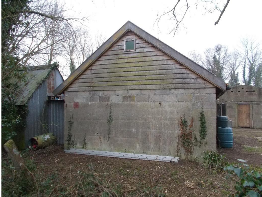
Photograph 1: North gable end
