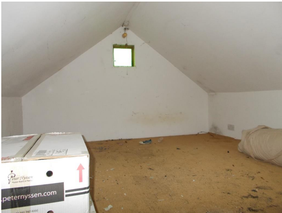
Photograph 8: Mezzanine / attic level
