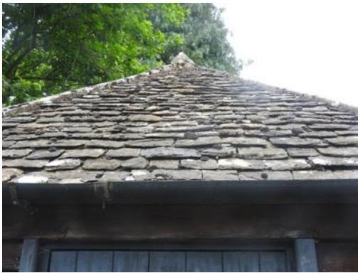
Figs. 27 & 28 Ridges and roof tiles of the hipped roof (L) north gable (R)
