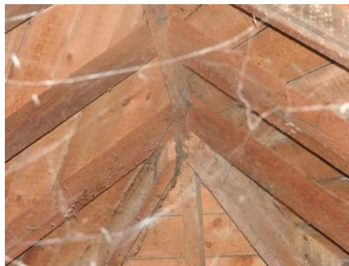
Fig. 33 Cobwebbed plumb cut
