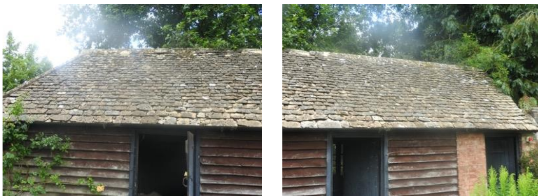
Figs. 23 & 24 Ridges and roof tiles to the east
