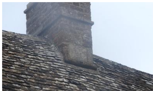
Figs. 13 & 14 Sealed chimney bases
