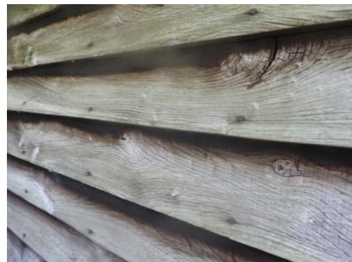
Figs. 29 & 30 Sealed eaves (L) and tightly fitting weather boards (R)
