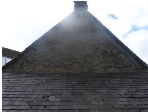
Fig. 17 Sealed gable to the north
