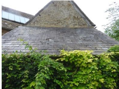
Fig. 12 Roof tiles of the mono-pitched garage
