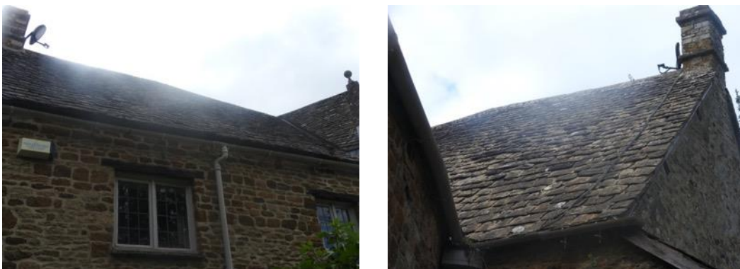
Figs. 6 & 7 Ridges and roof tiles to the northeast
