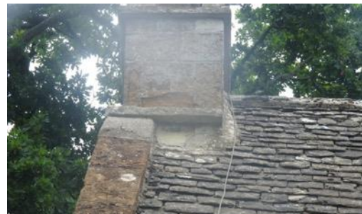
Figs. 13 & 14 Sealed chimney bases
