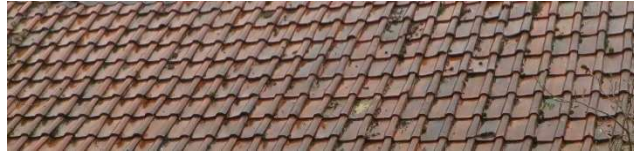
Handmade clay Roman pantiles to match existing outbuilding.
