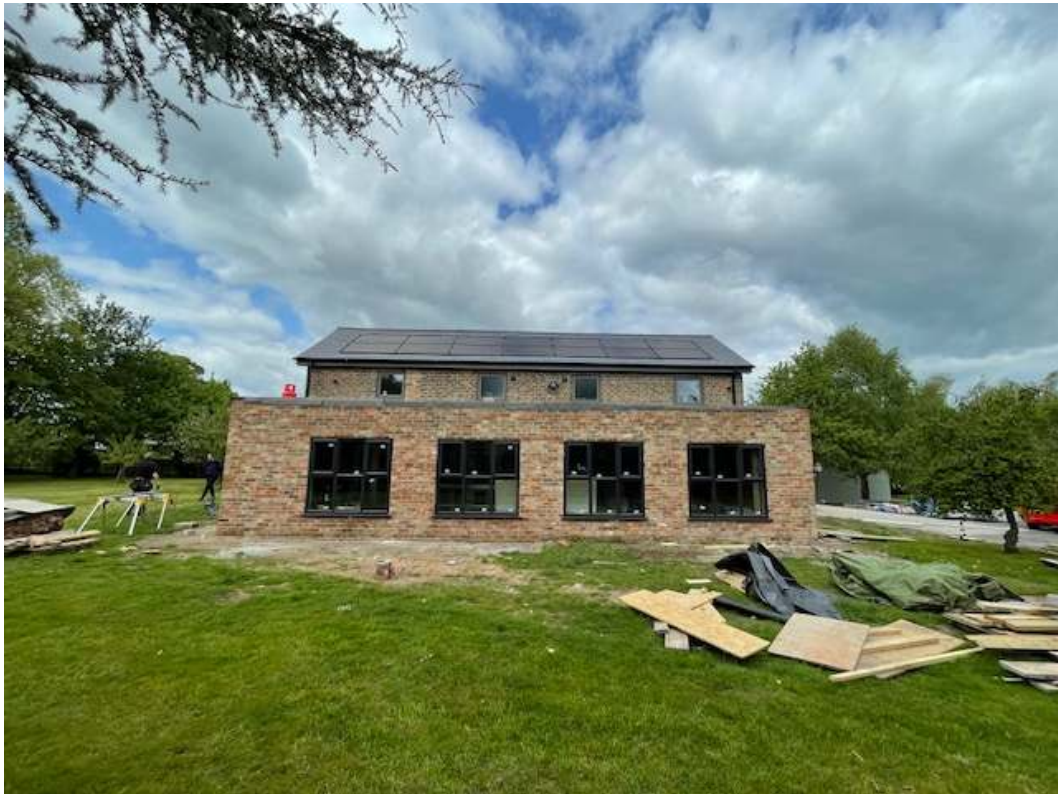
Image 6: Recent photograph of extension which is currently under construction
