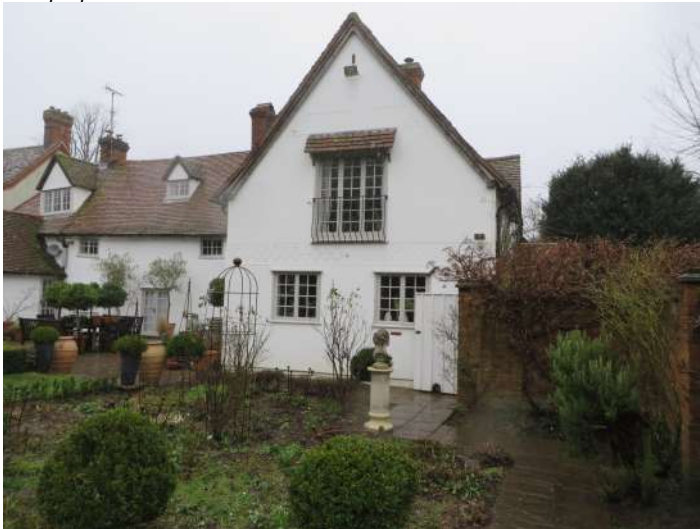
Two storey 1982 eastern cross wing extension at the rear
