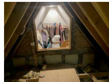
Hatch link to historic roof space
