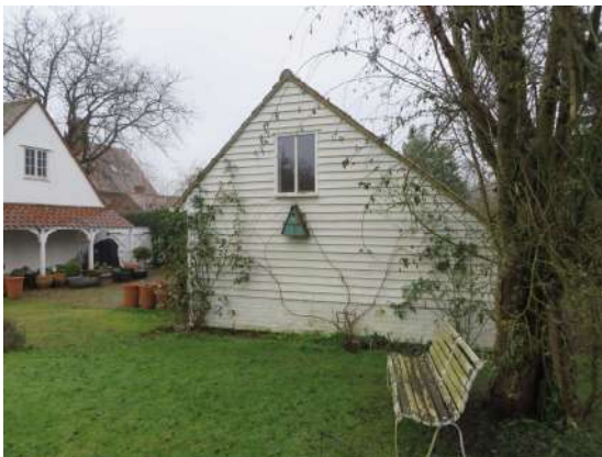
Existing annexe in foreground with 1982 garage beyond
