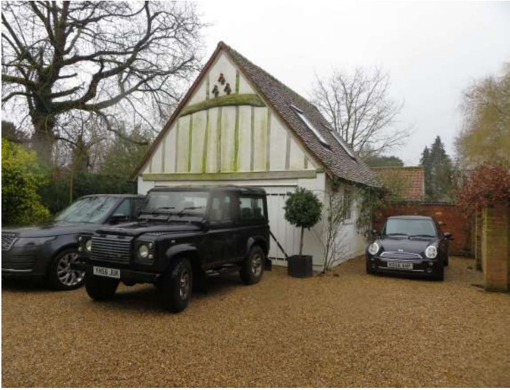
Garage is set at the back of the drive to the side of the 1982 eastern cross wing.
