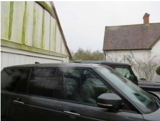
Garage sits to the side of the 1982 eastern cross wing.
