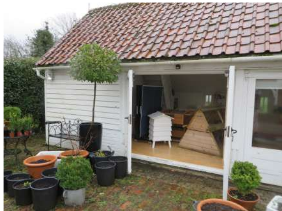
Existing annexe was previously a three-bay garage
