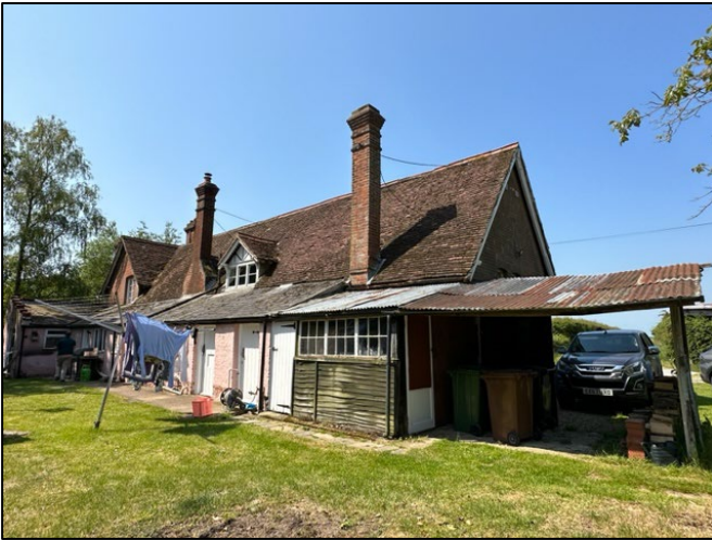
a) Extension, to be demolished and replaced.
