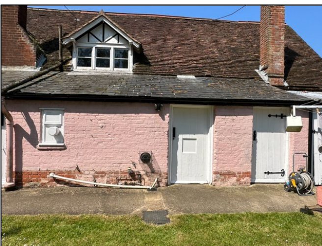
c) Store and utility room.
