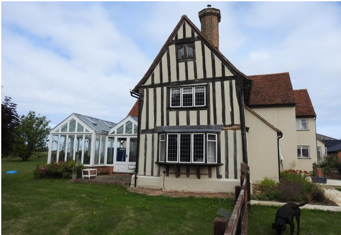
Illus. 2. The south-eastern gable, facing the Kersey road, with the remains of the medieval Wicker Street Green on the left. Until the 1960s the house consisted only of two wings adjoining at right-angles: the conservatory on the left and the projections to the right are modern additions. The gable windows are also modern (compare figure 11), and many of the associated timbers have been renewed. The chimney appears to survive from the 17 th century but has been heavily repointed.
