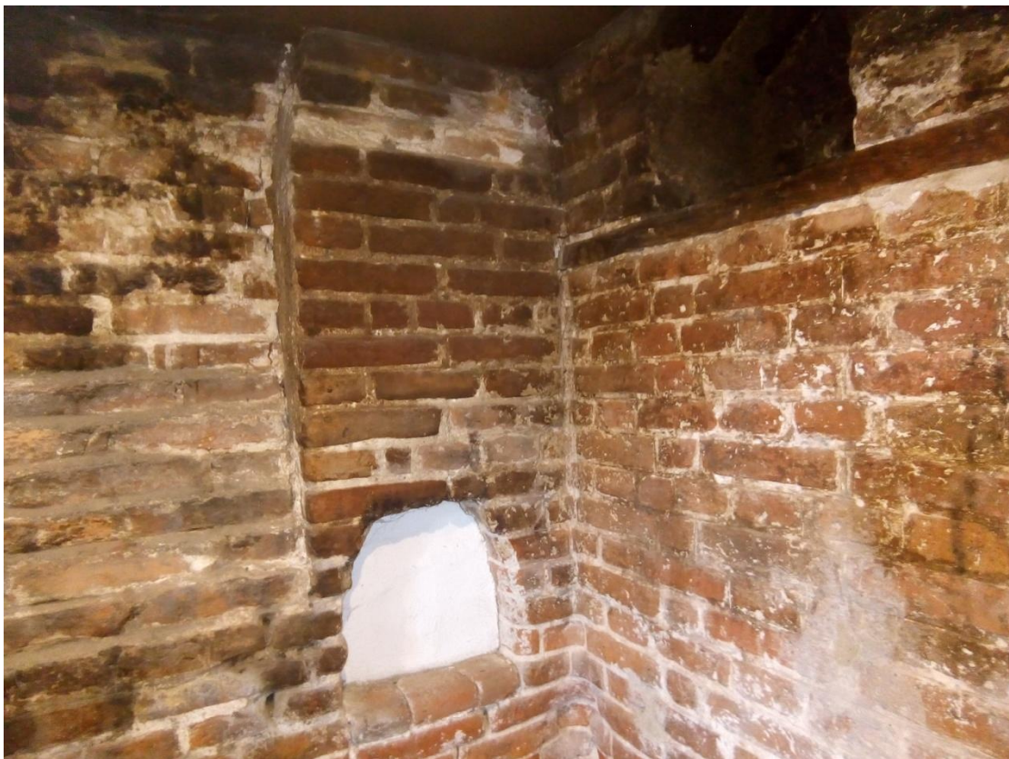
Illus. 12. The right-hand corner of the hall fireplace showing a pair of storage niches.
