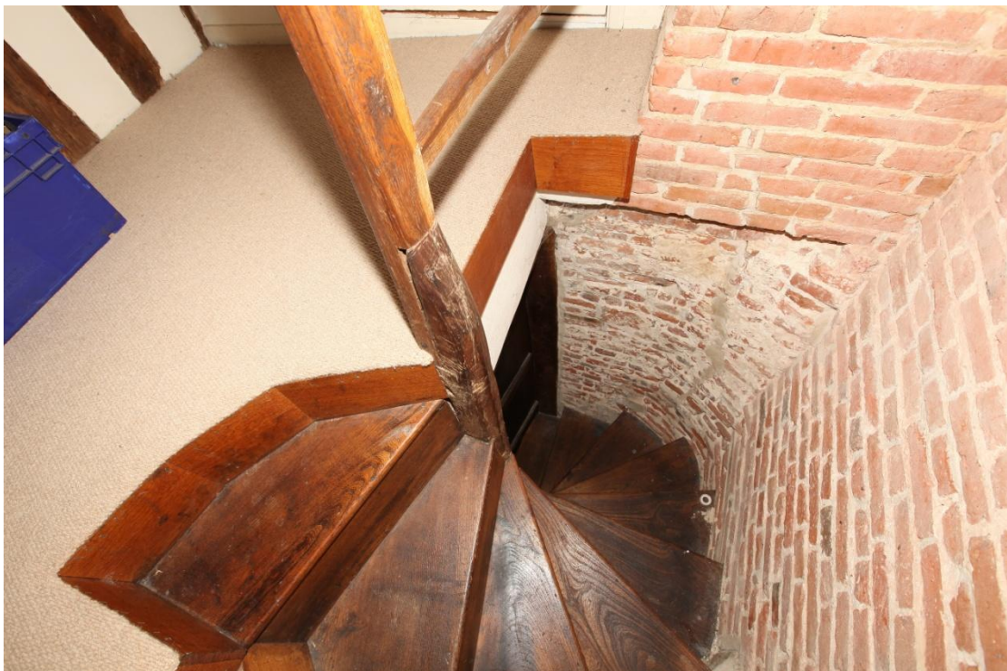
Illus. 24. The newel stair built into the south-western side of the chimney between the hall and parlour (as seen from the direction of the parlour chamber to the south-east). The lower section of the newel post appears to be original and while the tread-boards are modern they may conceal the original steps beneath. The stair and chimney may have been built when a ‘lobby entrance’ was inserted into the house, replacing the previous cross-passage.
