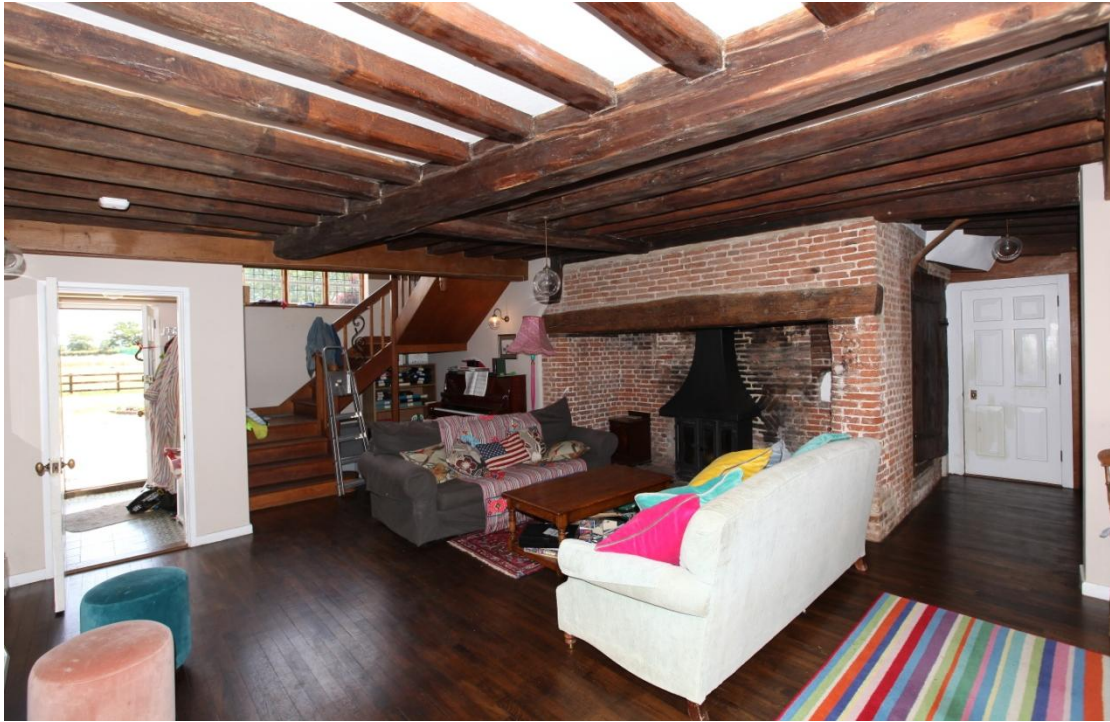
Illus. 9. The central hall from its western corner, showing the door to the parlour on the right. The north-eastern wall on the left was completely removed in the 1960s when the gabled extension containing the modern staircase was added. The ostensibly original boarded door to the 17 th century stair is visible in the side of the chimney (to the left of the parlour door). Note the scar of a missing partition on the ceiling joists at top left that may relate to a former cross-passage screen.
