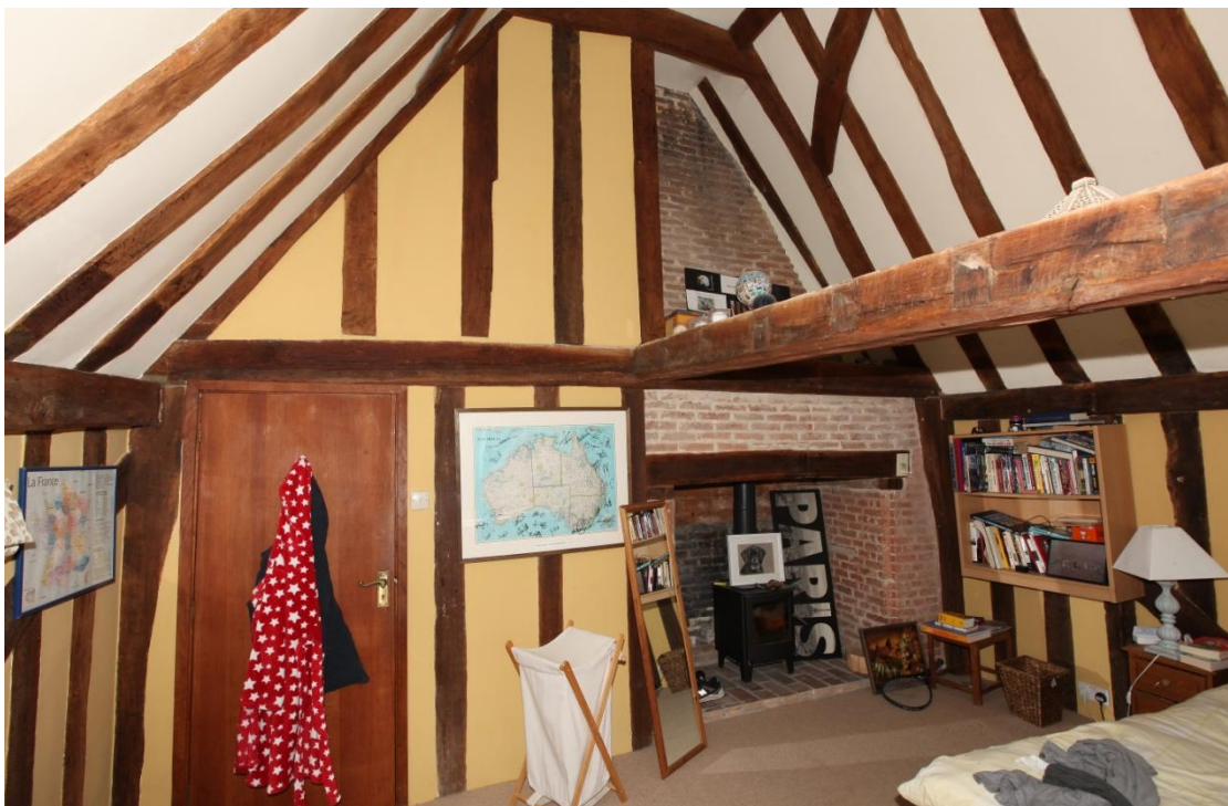
Illus. 22. The parlour chamber from its south-eastern gable showing the well preserved 17 th century fireplace above the ground-floor example in illus. 6. This too retains its original reddled finish. Note the empty mortices in the axial joist for the large, flat-sectioned common joists of a missing original ceiling. The principal rafter above the fireplace contains a pegged mortice for another curved wind-brace that projected into the chimney bay and was cut by the later brickwork of the present chimney.
