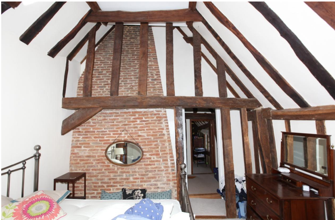
Illus. 14. The first-floor chamber above the central hall looking towards the chimney bay with the parlour chamber beyond. The studs to the right bear the diagonal weathering scar of the lower hall against which the chimney bay and parlour were originally built (illus 15). The diagonal timber to the left is an integral arch-brace rising from the truncated corner post shown in illus. 10 but the rest of the studs appear to be original despite the fact that they are nailed rather than tenoned to the frame. The clasped-purlin roof of the hall chamber lacks wind-braces but re-uses sooted rafters.
