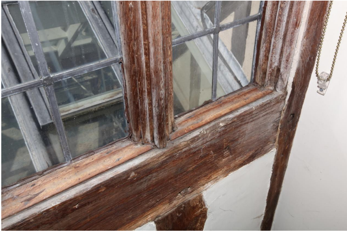
Illus. 19. A detail of the mullions in illus. 18. High-quality roll-moulded examples of this kind were fashionable in high-status buildings throughout the 16 th century but were quickly superseded by quarter-round ovolo mouldings at the turn of the 17 th . The later beading on the sill conceals small circular holes for saddle bars in the centre of each light to which leaded panels of glass would have been tied initially. These holes are still visible in the underside of the roof-plate above.
