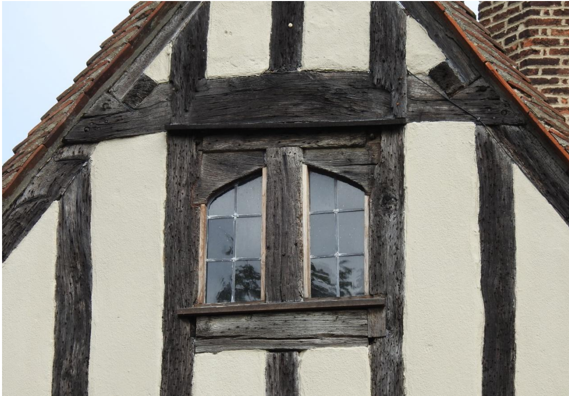
Illus. 3. A detail of the original arched attic-storey window in the south-eastern gable. The central stud is a later insertion. Arched 16 th century windows are usually found only in shop facades and examples at this height are rare. A close parallel of the same late-16 th century date can be seen nearby at 4 Nayland Road in Bures (figure 10).
