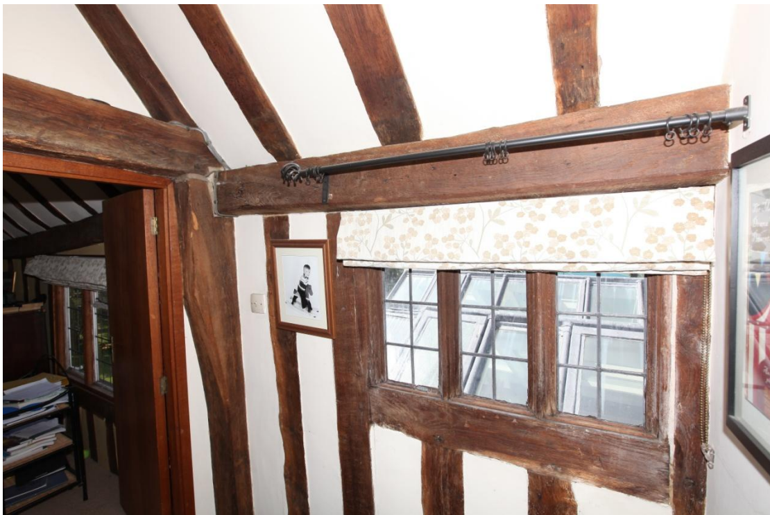
Illus. 18. The fine original window of roll-moulded mullions in the south-western facade of the chimney bay with the parlour chamber on the left.
