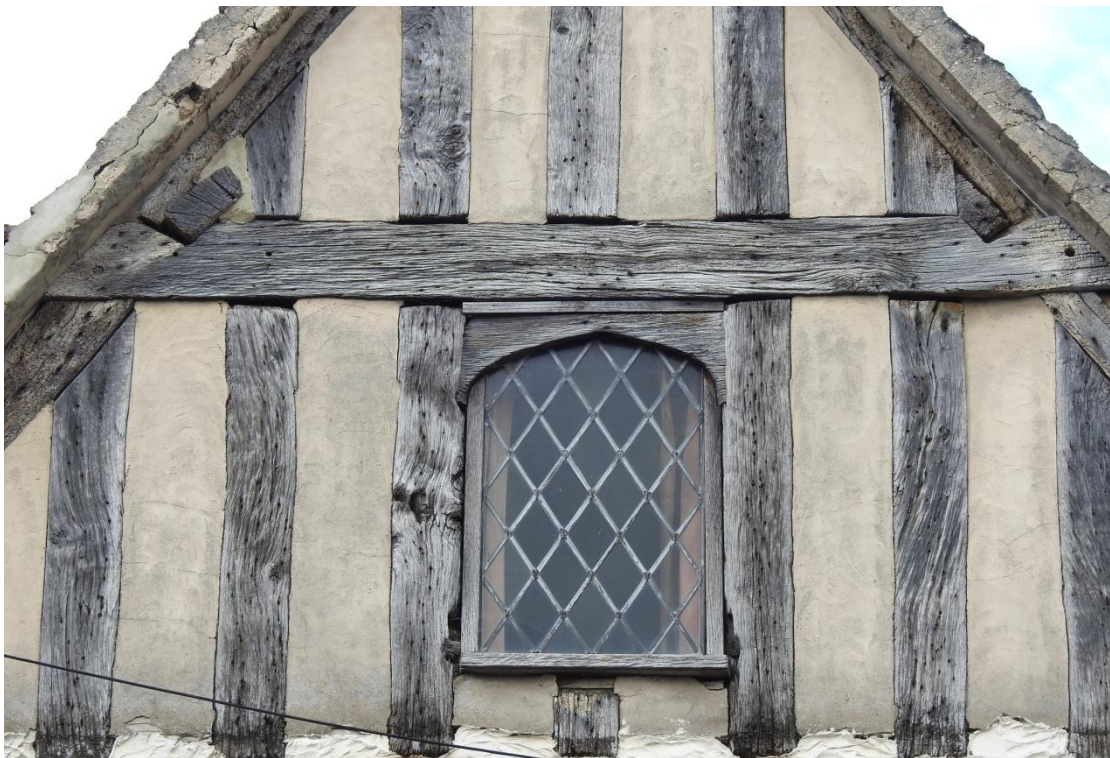
Figure 10. The identical arched gable window at 4 Nayland Road in Bures (illus. 3). Gable windows of this kind are very rare and as the rest of the framing is strikingly similar to that of Curtis Farm it was probably the work of the same carpenter. The Bures example lit a first-floor room without a ceiling.
