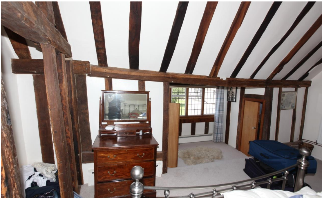
Illus. 16. The front (south-western) wall of the hall chamber showing its intact roof-plate with original studs and mid-rails on each side of a central aperture cut to link the chamber with the lean-to extension of the 1960s. These studs are widely spaced relative to those of the parlour but are weathered externally and were evidently exposed.
