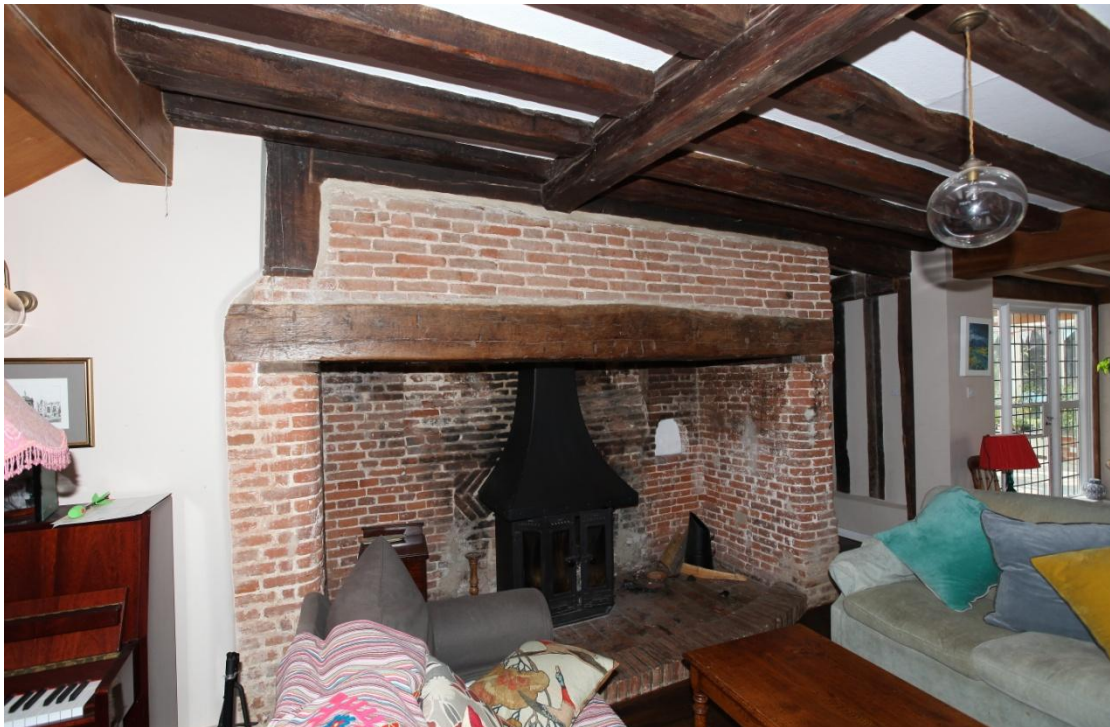
Illus. 10. Like its counterpart in the parlour the hall fireplace survives largely unaltered from the 17 th century but the timber frame was built for a smaller, earlier chimney and the fireplace cuts the corner post on the left. Note that the axial joist of the ceiling is central to the wider hall and not the binding joist above the chimney.
