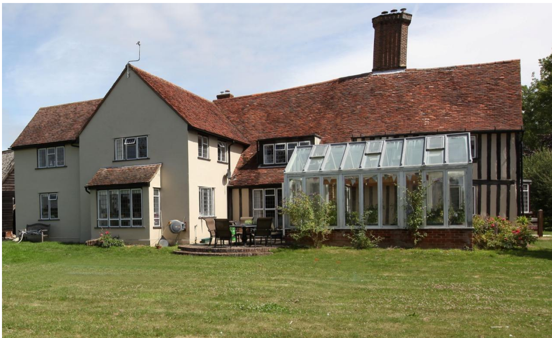
Illus. 4. The original south-western facade, seen from the medieval green. Compare the photograph of the same elevation in 1959 (figure 11). The red-brick fabric of the left-hand wing has been disguised with cement render. The lean-to in the angle of the two historic wings was added in or about the 1960s while the glazed conservatory and the two-storied projection on the left date from 1992 and 1994 respectively. The original first-floor window with moulded mullions in illus. 18 is hidden behind the conservatory.
