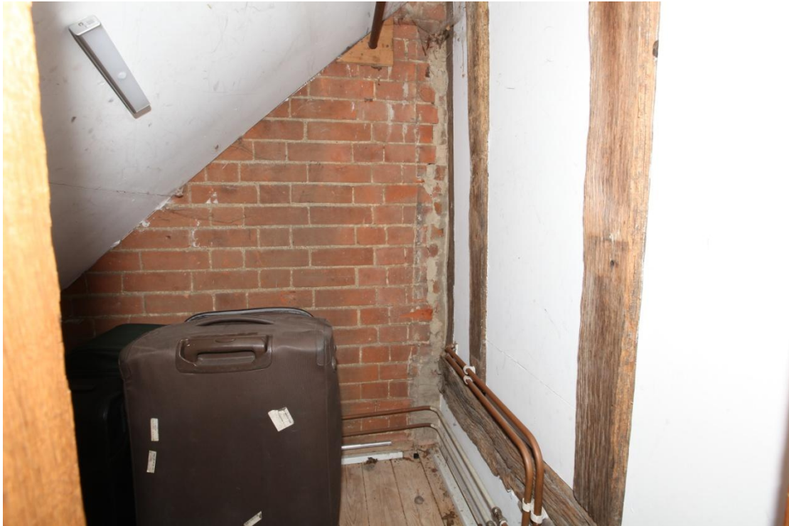
Illus. 17. The interior of the cupboard within the roof of the lean-to extension shown to the right in illus. 16. The red-brick fabric of the service cross-wing is visible to the left with the weathered studs and mid-rail of the original south-western facade on the right.
