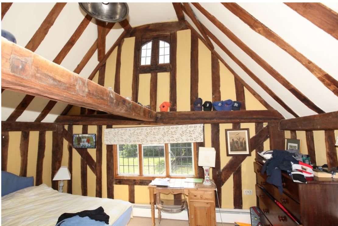
Illus. 20. The south-eastern internal gable of the parlour chamber showing its heavy frame with internally trenched braces and arched window. The axial joist on the left is tenoned and pegged to the tie-beams at both ends and is evidently an original feature.
