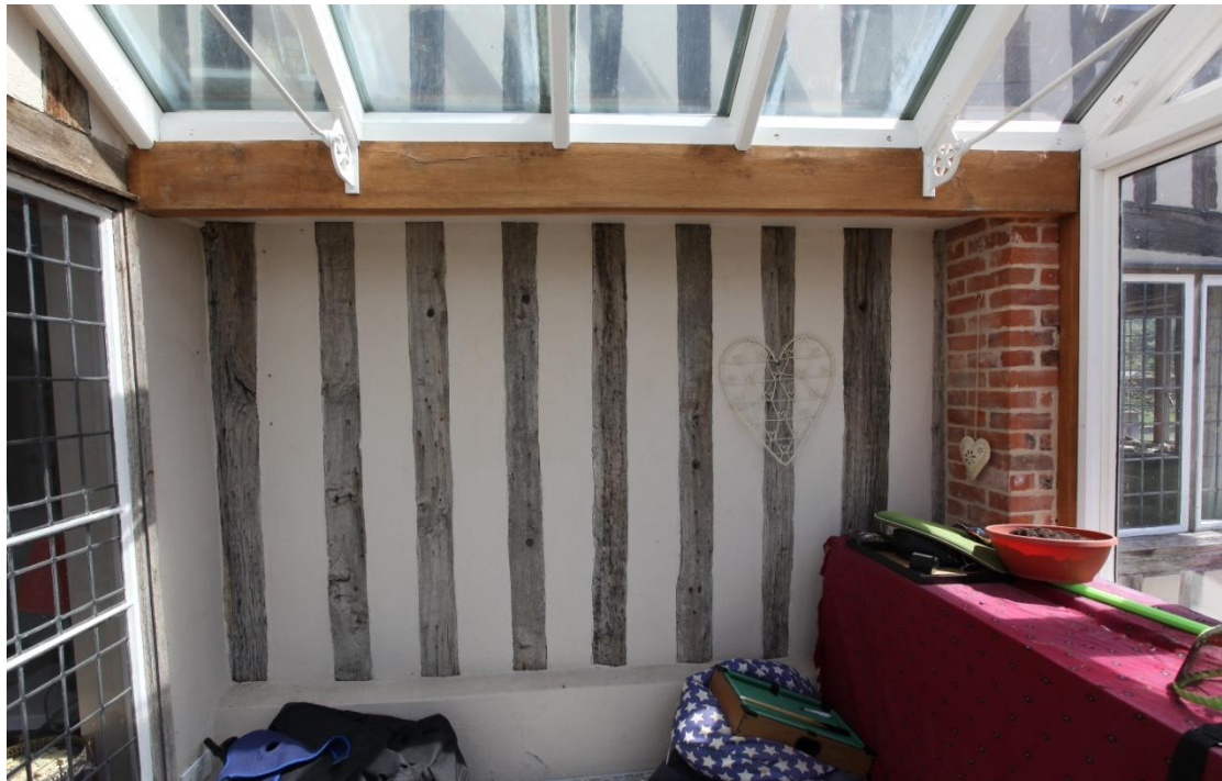
Illus. 5. The studs of the south-western facade from the conservatory which was initially added in 1992. The 1959 photograph shows a ‘lobby entrance’ door in this position, and the central two studs are insertions that are not pegged to the mid-rail – suggesting the door was either an original feature or more probably occupied the position of an original window. The weathered storey posts of the chimney bay are visible to left and right but all six central studs lack weathering and are recent replacements.
