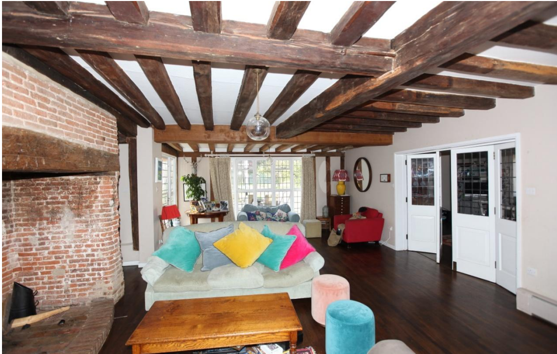
Illus. 11. The central hall from the north-east, with the 20 th century folding doors to the brick service wing on the right. The original front wall facing the green lay beneath the light-coloured modern ceiling beam in the background but was entirely removed on the ground floor when the lean-to extension was added beyond. The joists and wall studs of this extension are modern.
