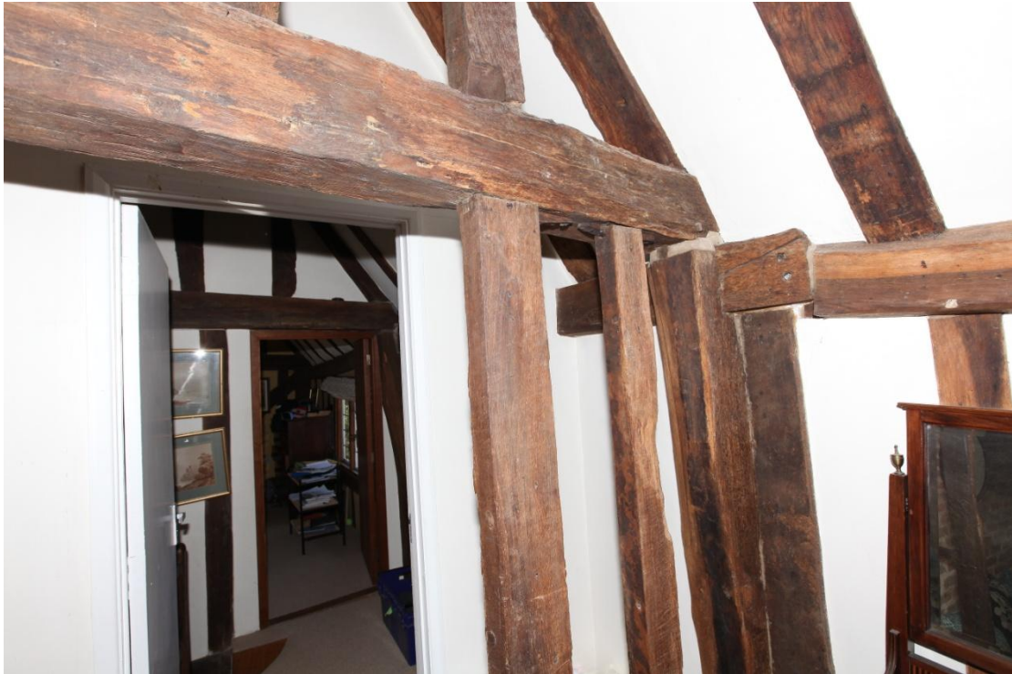
Illus. 15. A detail of the framing to the right in illus. 14. The frame of the hall chamber is a 17 th century replacement of a lower predecessor that almost certainly represented a medieval open hall. Its roof-plate at top right is lapped and pegged to the end of the late-16 th century parlour roof-plate which is clearly weathered where it once projected above the medieval roof. The angle of this medieval roof is reflected by a diagonal weathering scar to the tie-beam and wall studs, with those at top-right once exposed while the area to the left was protected with the missing roof and remains unweathered.
