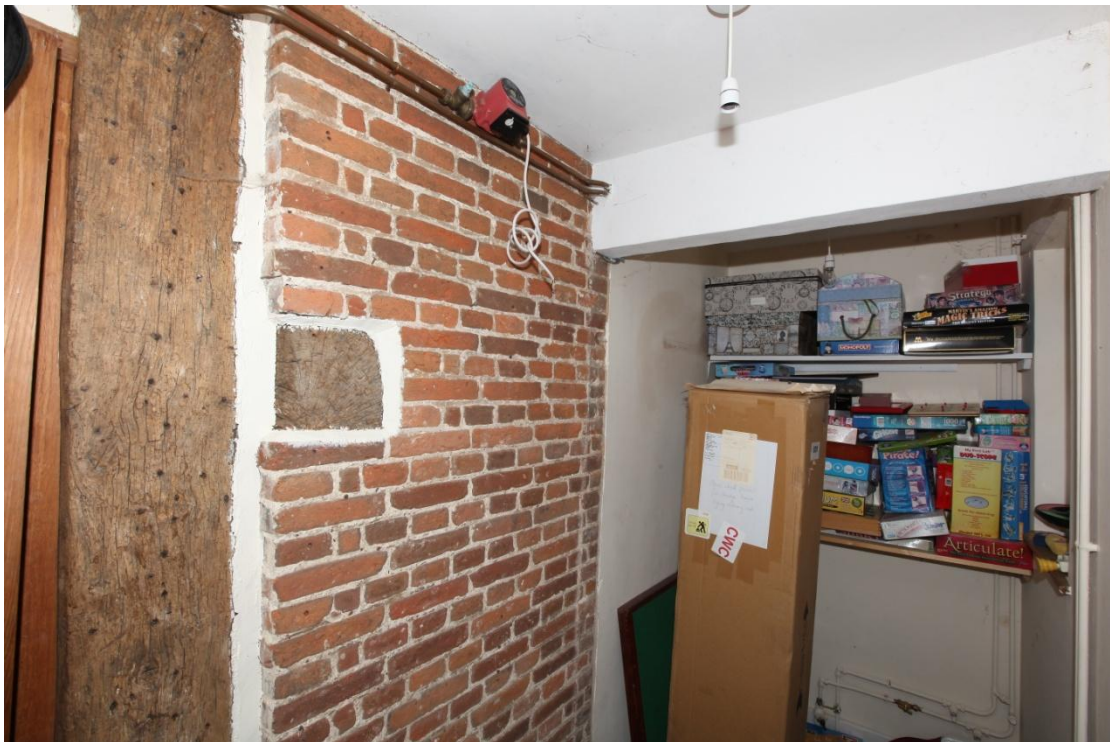
Illus. 8. The north-eastern side of the brick chimney with the corner-post of the parlour on the left. The lintel and brickwork project through the timber-framed wall and are weathered, having been exposed to the elements until the addition of the lean-to in the 1960s. This unusual feature demonstrates that the present chimney post-dates the frame.
