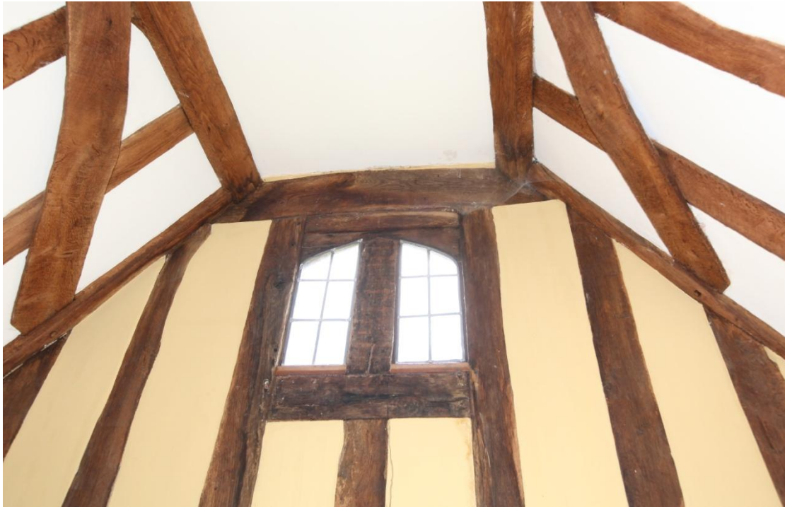
Illus. 21. A detail of the rare arched window in the roof gable of the parlour. This appears to have lit an attic chamber as there is evidence of a missing original ceiling in the chamber beneath, although in other respects the framing is identical to that of 4 Nayland Road in Bures which lacked an attic floor.
