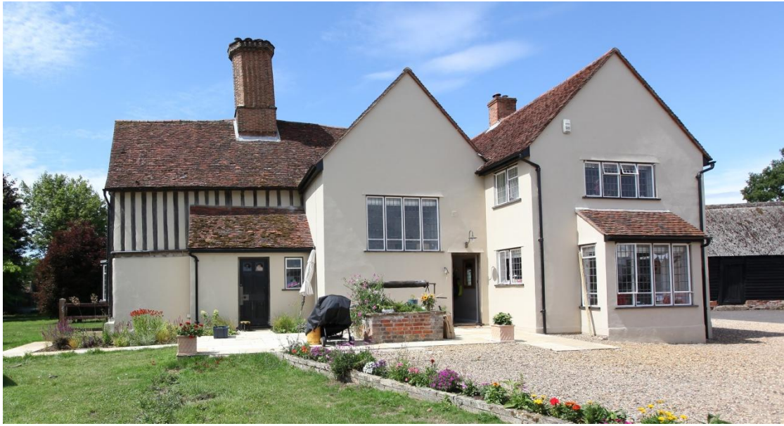
Illus. 1. The house from the present entrance to the west with the impressive 17 th century ‘concertina’ chimney between the hall and parlour on the left. This was the rear elevation of the house until an extensive renovation in the 1960s which saw the addition of the lean-to against the chimney and both gabled projections to the right.
