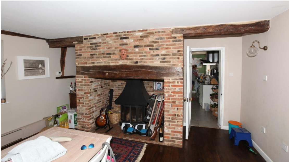
Illus. 13. The fireplace against the rear (north-eastern) gable of the original service wing. The modern kitchen beyond is an extension of the 1960s. The 19 th century Ordnance Surveys show what appears to be an external chimney projecting from this gable but the present fireplace is a 20 th century reconstruction that re-uses an early lintel. Some of the adjoining timber may be in situ but most has also been re-used. The rest of the wall fabric in the wing is hidden by modern render but appears to be of brick.
