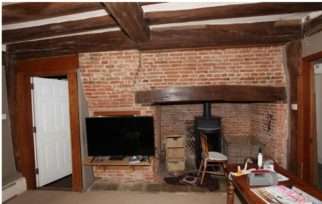
Illus. 6. The good 17 th century fireplace in the heavily timbered late-16 th century parlour with the projection of the integral staircase to the left of the lintel. Although the brickwork occupies a dedicated narrow chimney bay it projects through the original external wall on the right and is clearly a replacement of the narrower stack for which the frame was designed. A number of ‘taper’ burns are visible on the lintel.
