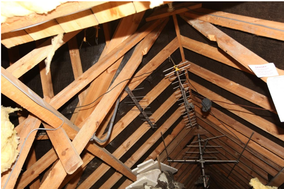
Illus. 26. The softwood roof of the brick service wing, rebuilt either as part of the 1960s restoration or when the wing was extended in the early 1990s. Re-used sooted rafters that were probably salvaged from the medieval open hall on the site are visible in the roof of the hall range to the left.
