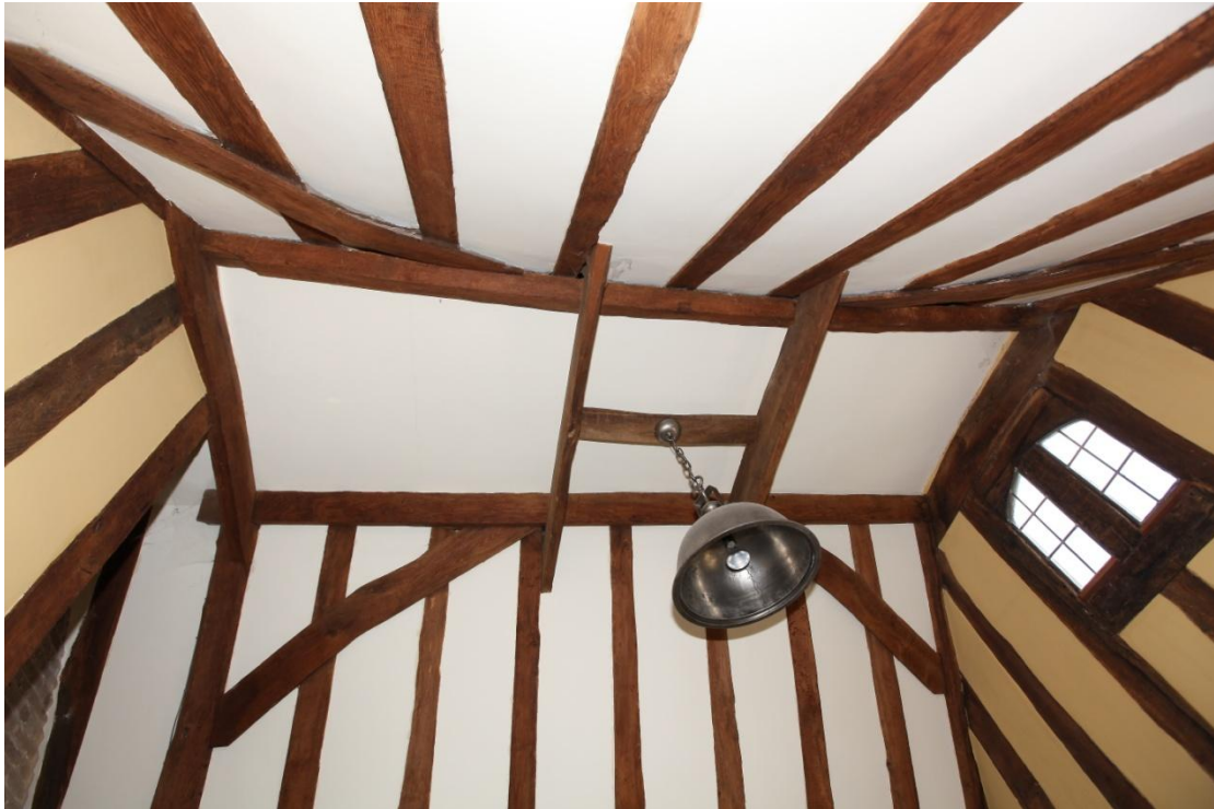
Illus. 25. The clasped-purlin roof of the parlour bay showing its curved wind-braces in the typical style of the mid- and late-16 th century. The purlins and braces continued into the chimney bay on the left but were cut when the chimney was rebuilt. The hall roof is also of clasped-purlin form but lacks wind-braces and contains a number of re-used rafters including several heavily sooted examples salvaged from a medieval open hall.
