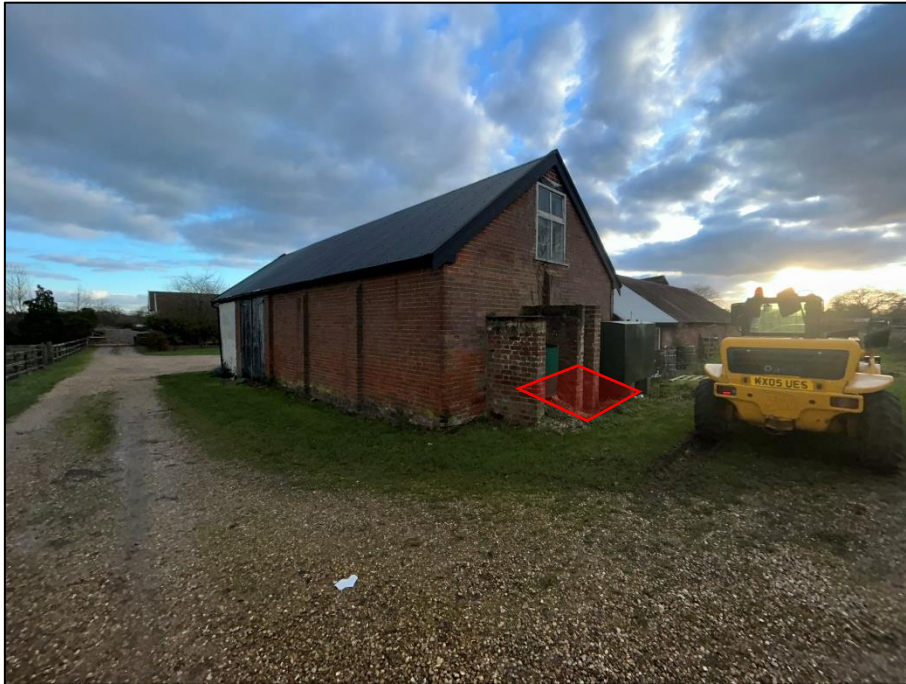
Photograph 11 – Extension of external excavation
