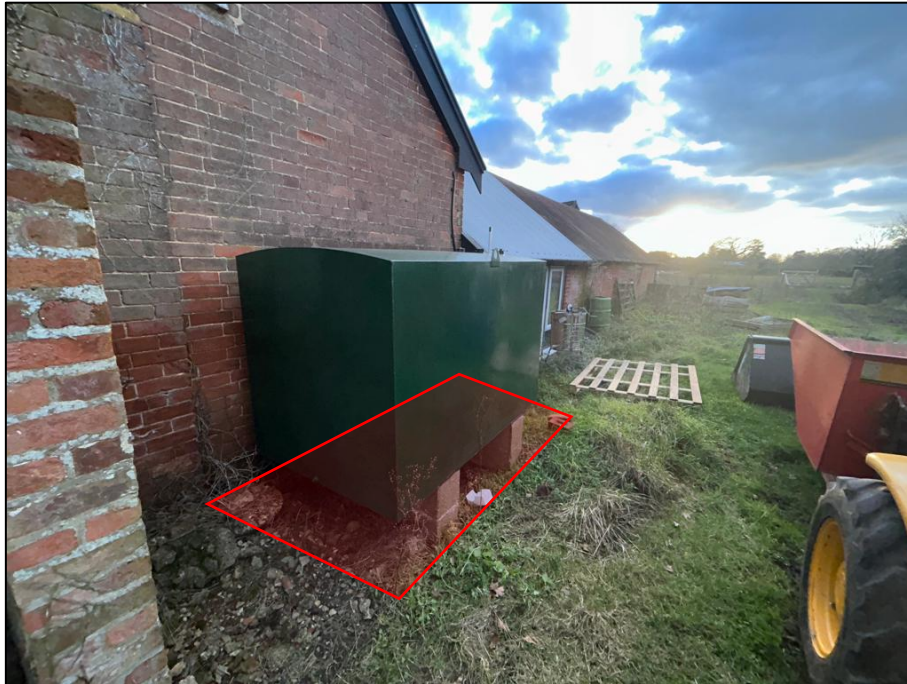
Photograph 9 –View of tank location
