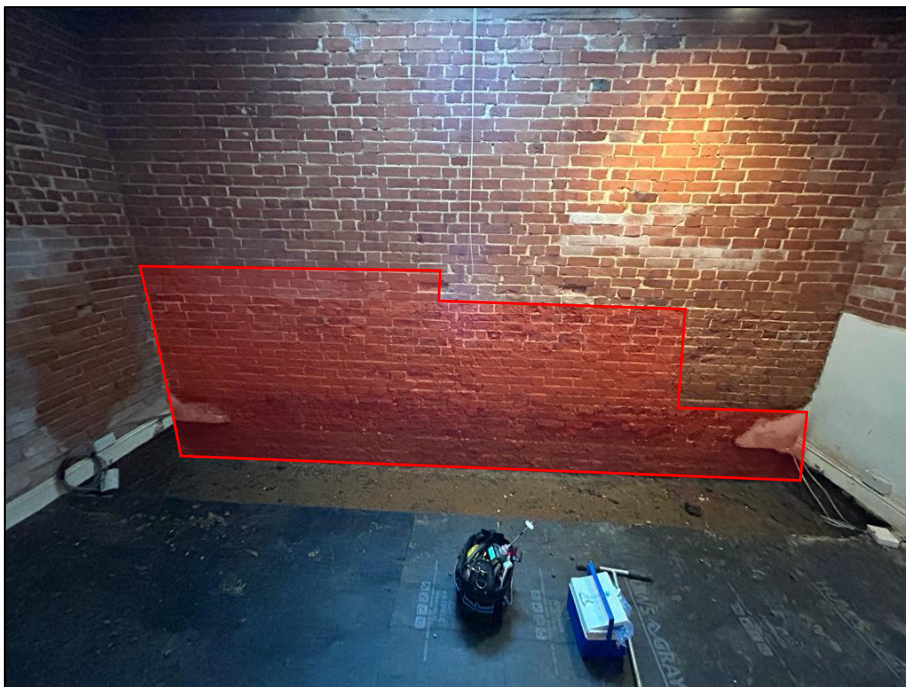
Photograph 12 – Internal brickwork replacement
