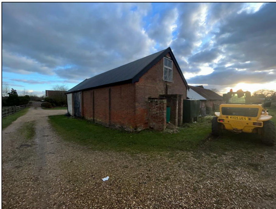
Photograph 8 – Track to external works area
