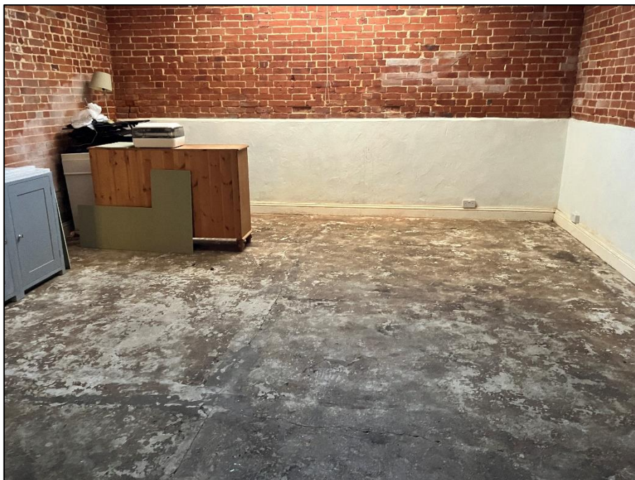
Photograph 6 – View of internal works area
