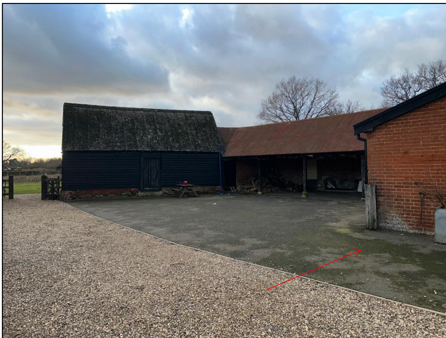
Photograph 4 – Front aspect of outbuildings / works area with possible skip location
