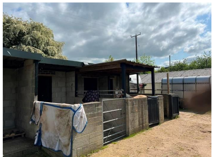
Outbuildings to southeast of application site
