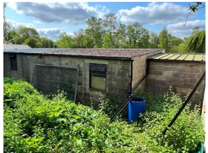
Northeast and northwest elevations of southeast outbuilding and store
