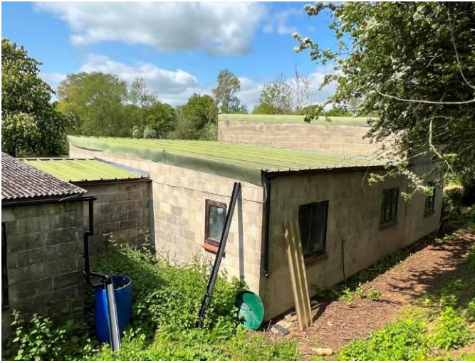
Northeast and northwest elevations of northwest building
