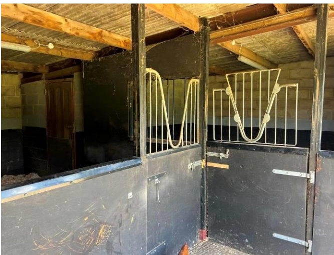
Interior of southeast outbuilding
