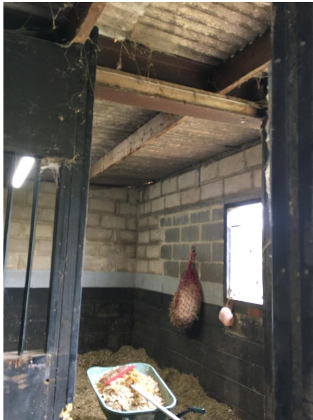
Photograph 10 Stables – Steel beam supporting timber roof joists
