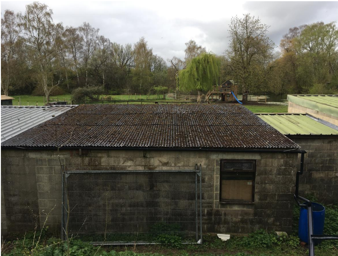
Photograph 4 Stable Block – Rear elevation and roof
