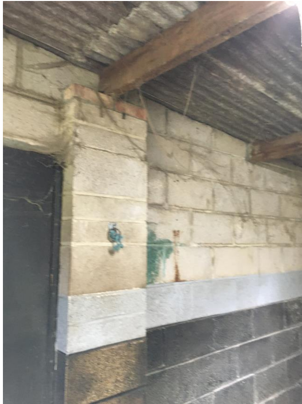
Photograph 9 Stables – Stiffening pier
