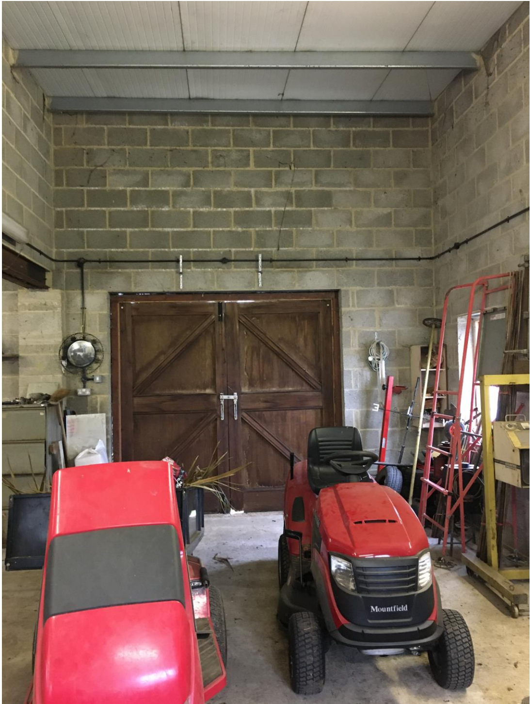
Photograph 15 Workshop - Blockwork inner leaf
