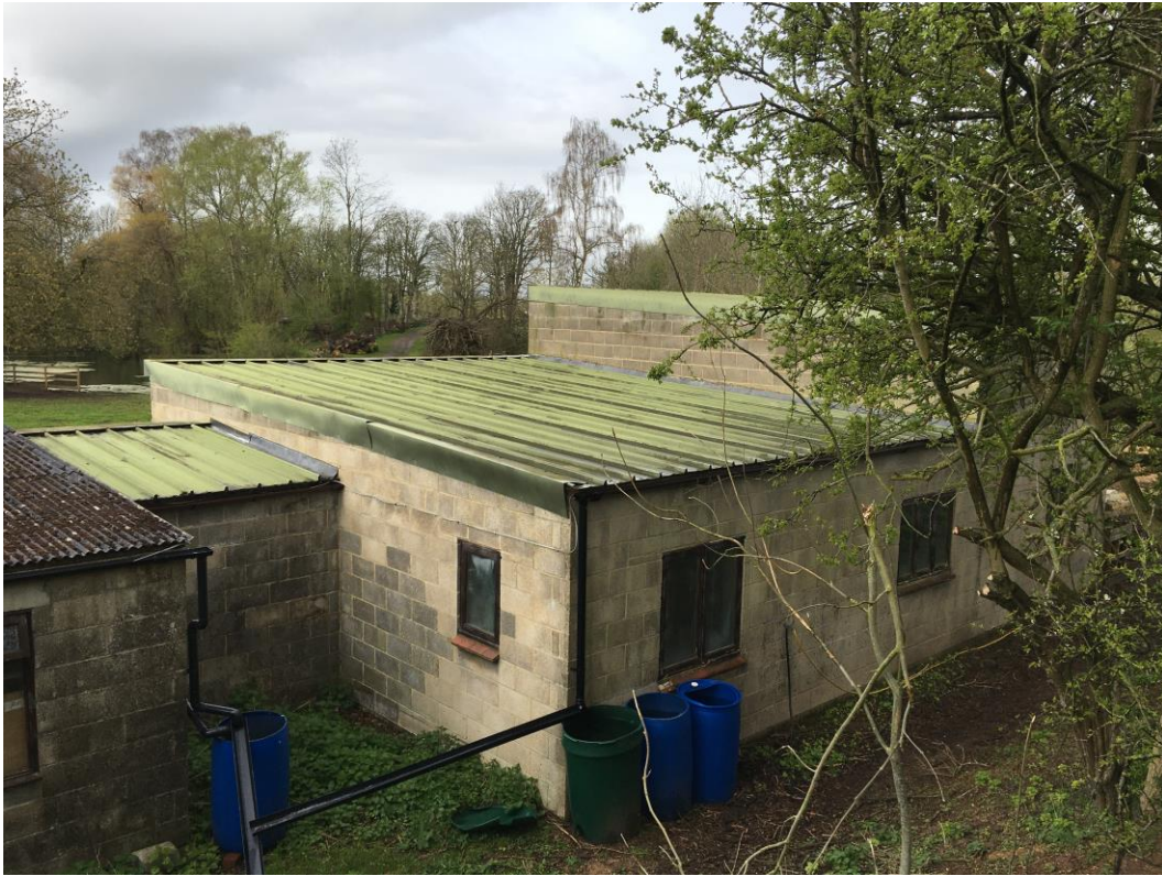
Photograph 3 Workshop and Store – Rear and side elevations and roof
