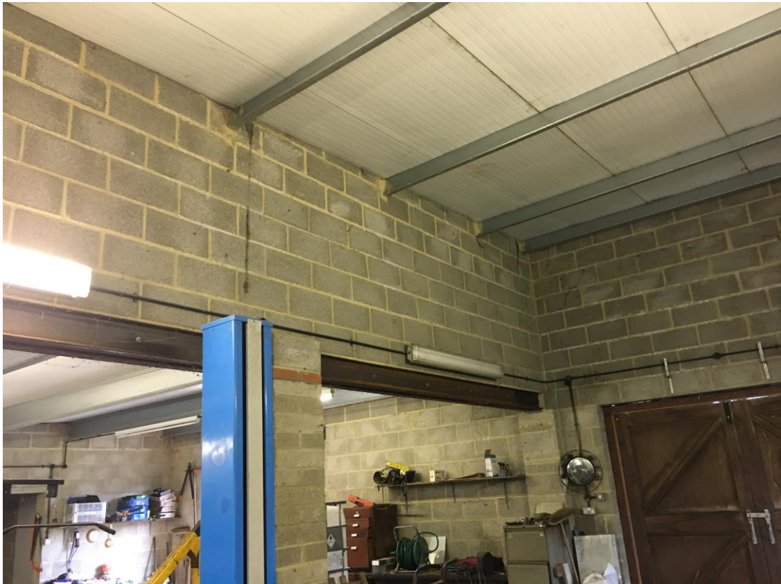
Photograph 14 Workshop higher level roof
