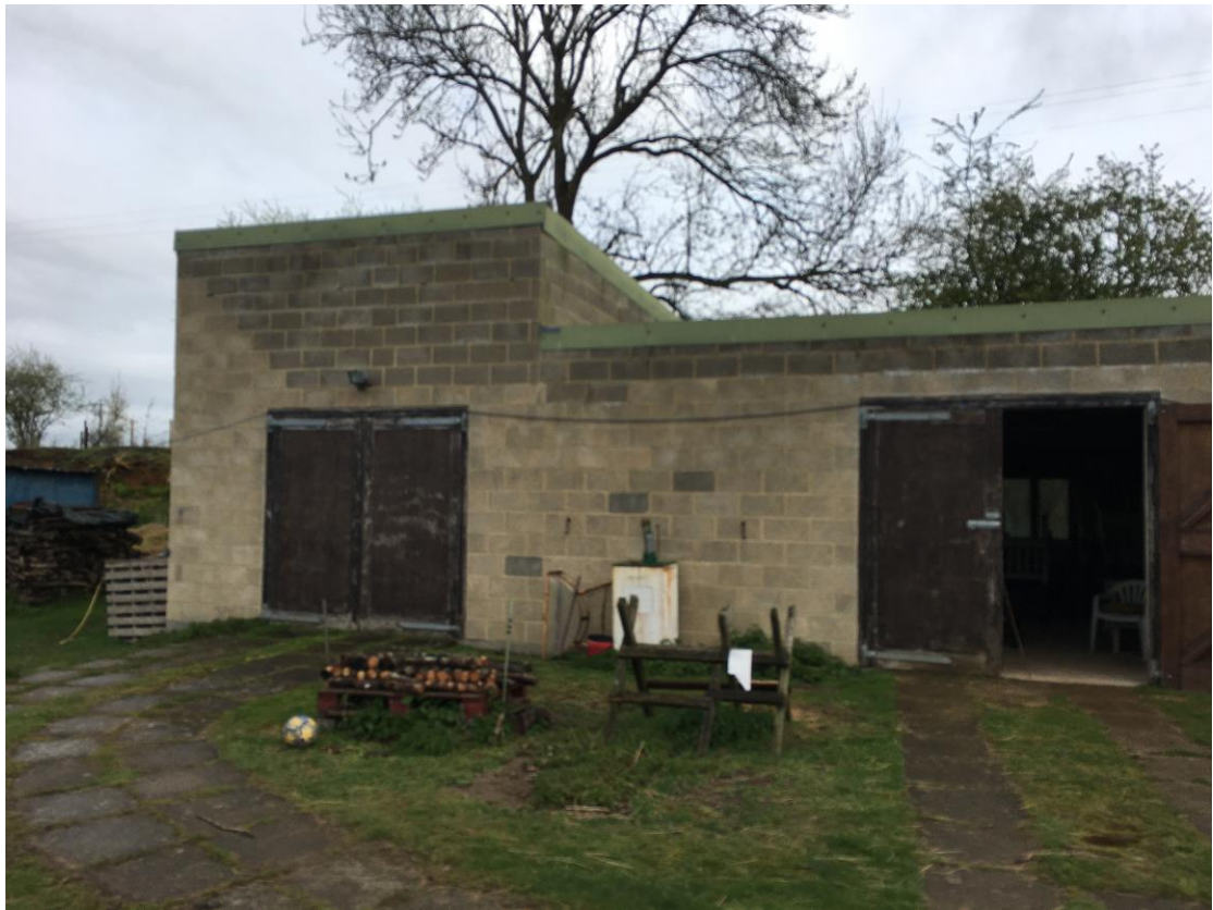
Photograph 1 Workshop Front elevation
