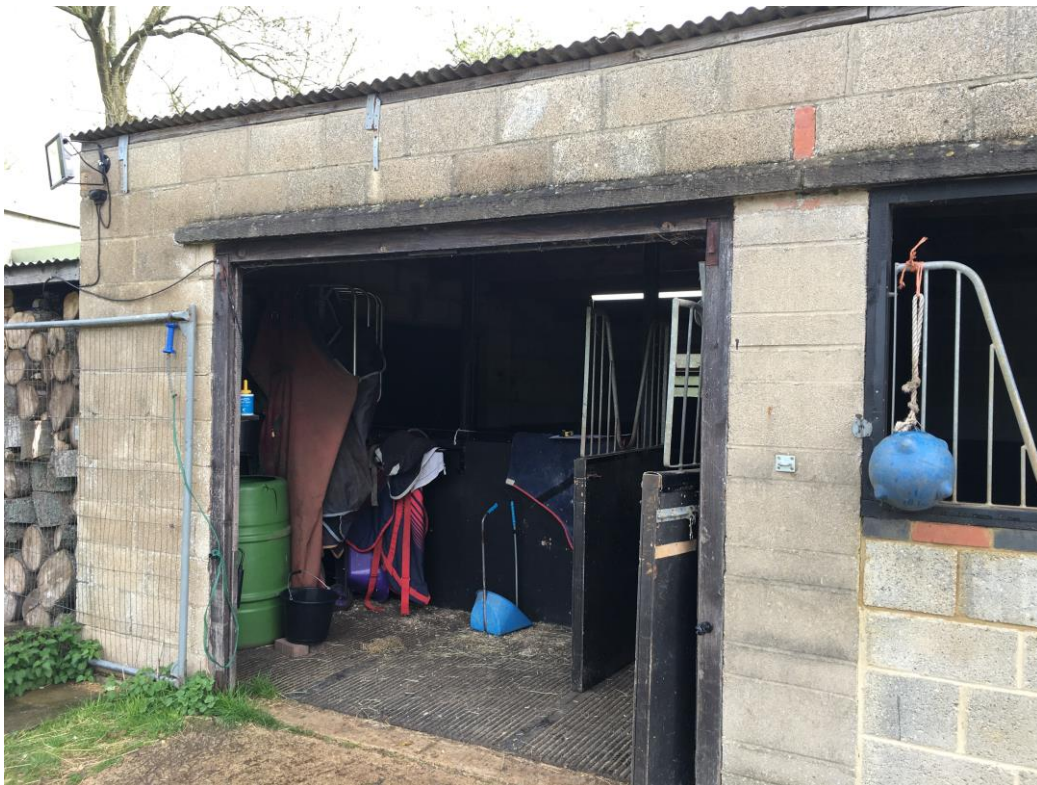
Photograph 8 Stables – Precast concrete lintel over door
