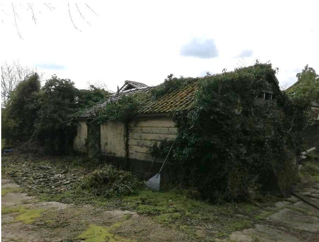
Photograph 4: Timber cladding and clay-lump barn with pantile roof and ivy
