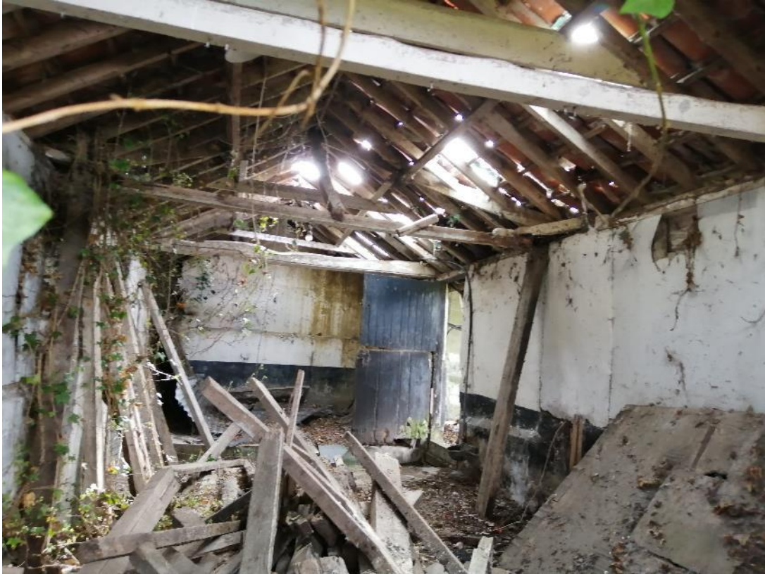
Photograph 5: Interior of timber cladding and clay-lump barn with pantile roof
