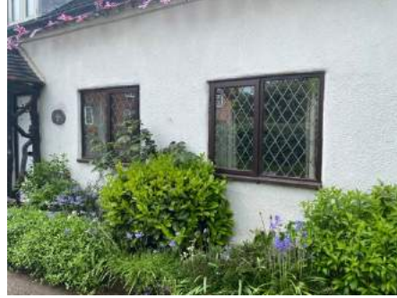
EXISTING WINDOWS (GROUND FLOOR)
