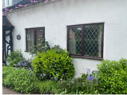
EXISTING WINDOWS (GROUND FLOOR)
