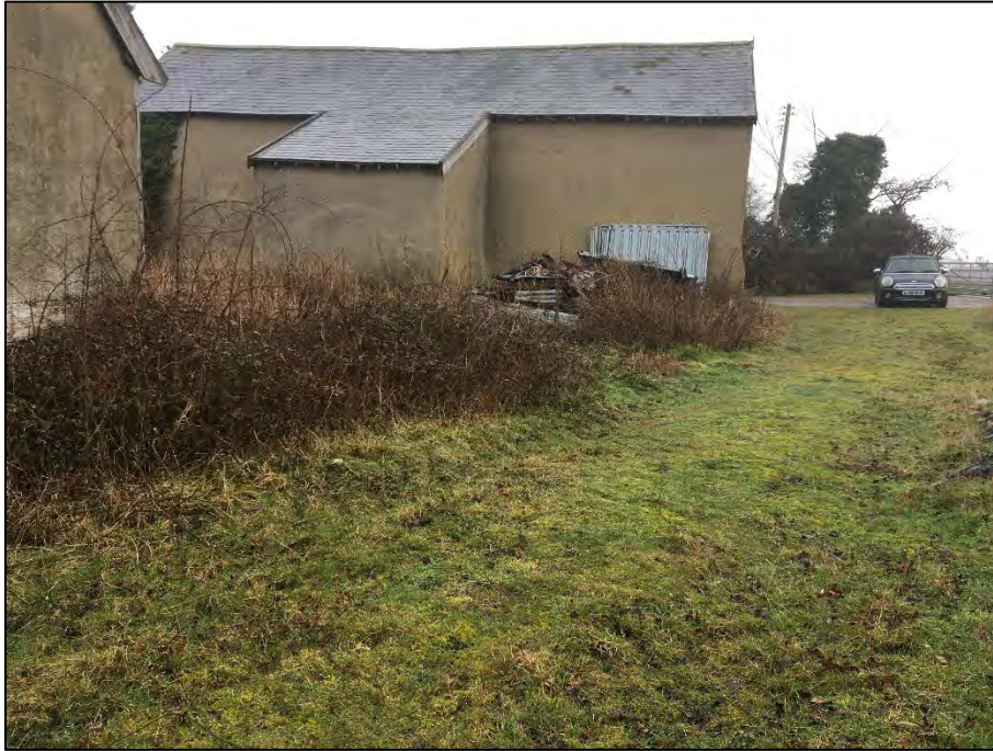
Photograph 27: The farm building close to the site entrance, which was in use for storage.
