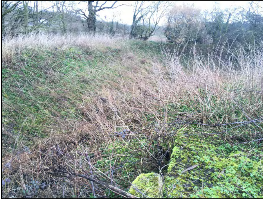
Photograph 9: The deep and large dry pond to the east of the site.
