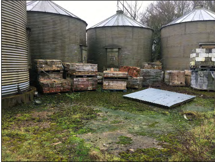
Photograph 31: The grain silos located in the south-western corner of the site. The metal sheeting was covering a water-filled hole in the ground.
