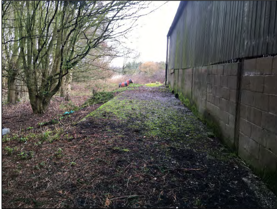
Photograph 7: The northern side of the large farm building in the eastern sector.
