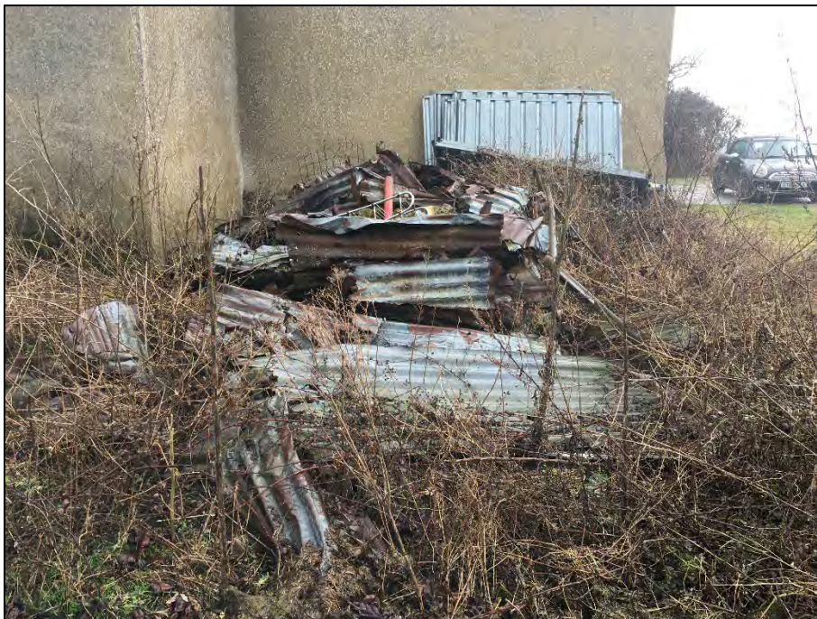
Photograph 28: Metal sheeting etc. to the rear of the building shown in Photograph 27.
