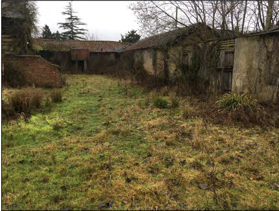
Photograph 19: The north-western sector of the site. The buildings were inaccessible from the site and were in use by the farmhouse located immediately to the north-west.
