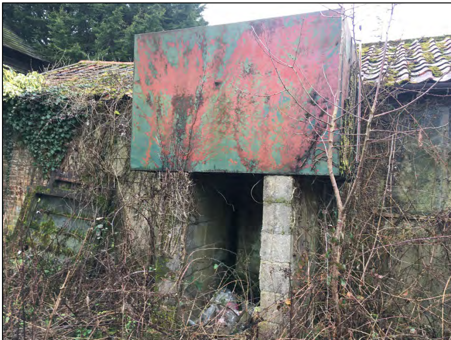
Photograph 20: The above ground fuel storage tank in the north-western corner.
