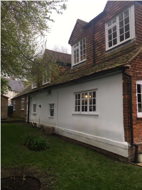
Existing rear Elevation with dormers added in the 1980's.
