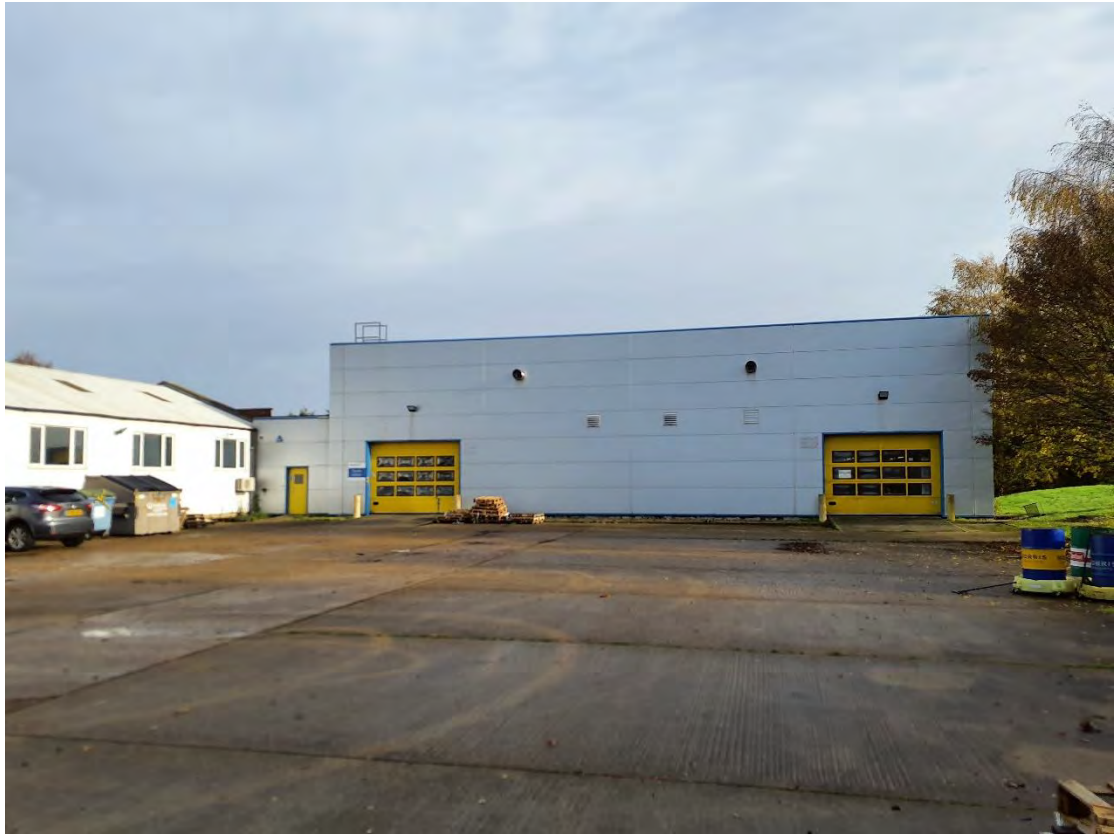
Figure 8 – Looking east at the main building from the south of the site.
