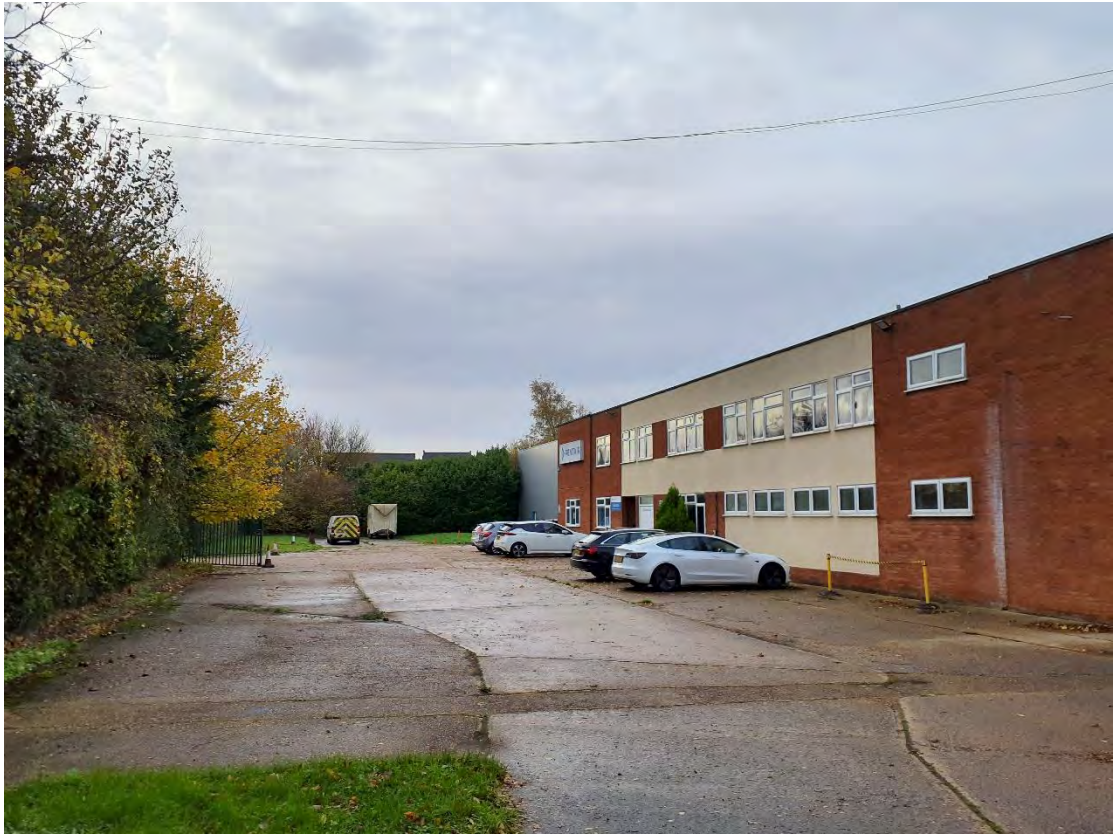
Figure 2 – Looking south down the site at the main building.
