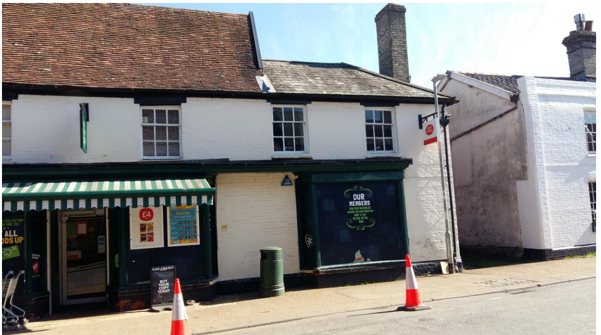
Front elevation to The Street, southeast end
