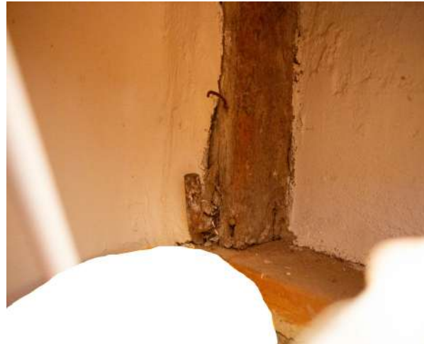
Fig 3.6 Historic metal hinge in Larder of No.4 suggesting existence of old doorway between No 4&6 previously before subdivision of property.
