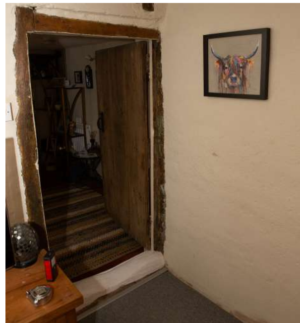
Fig 3.3 Living Room of No 6 showing doorway and ledged door leaf to be referenced in the new doorway design.
