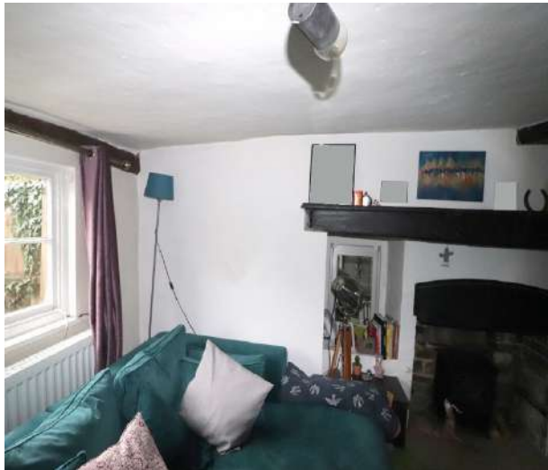
Fig 3.0 Location of Proposed Ground Floor Doorway from No 6 Living Room. [photo from HIA - Hoggett]
