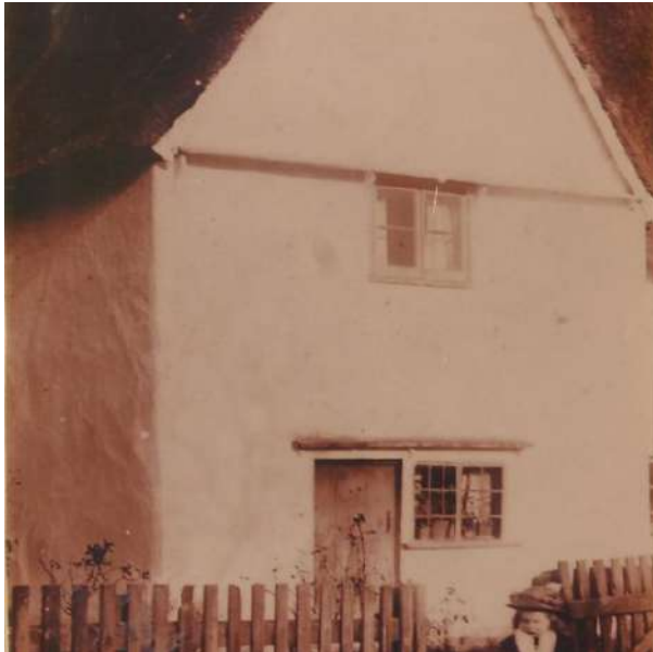
Fig 1.10 No 6. Photo in 1912 showing previous lime render external finish without roughcasting.
