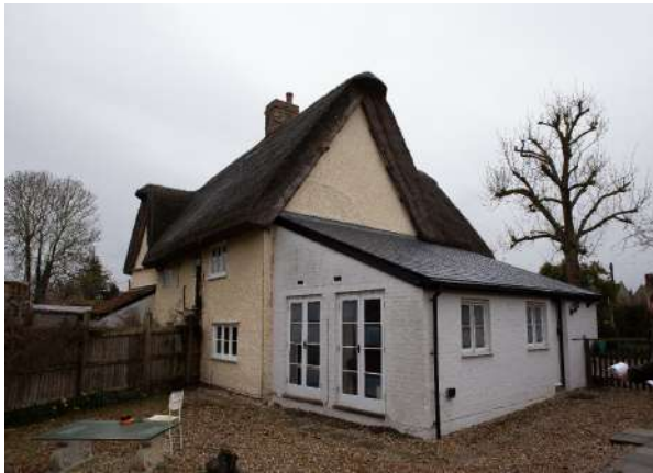
Fig 1.1 View of No 6 from North-West
