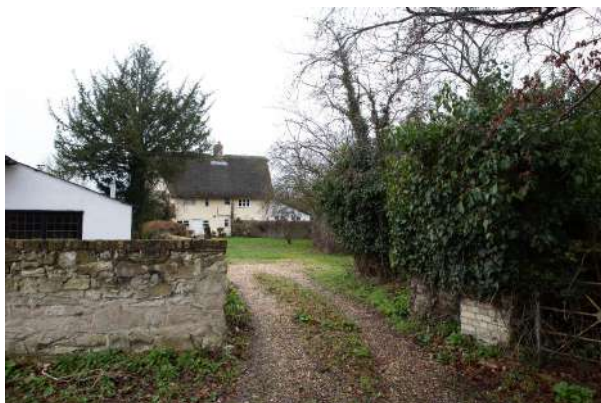
Fig 1.2 Rear/North elevation from Broad Lane and rear driveway entrance into garden of No 4
