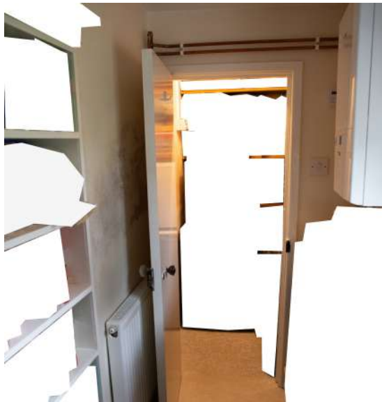
Fig 3.1. Larder to no.4 from Kitchen showing doorway and partition to be removed and wall where new doorway to go straight ahead. Belongings obscured.
