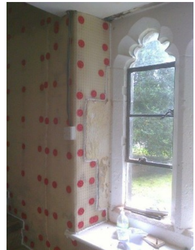
RUK Slimline used as a salt barrier in an historic building. Stone dressings to windows left exposed.
