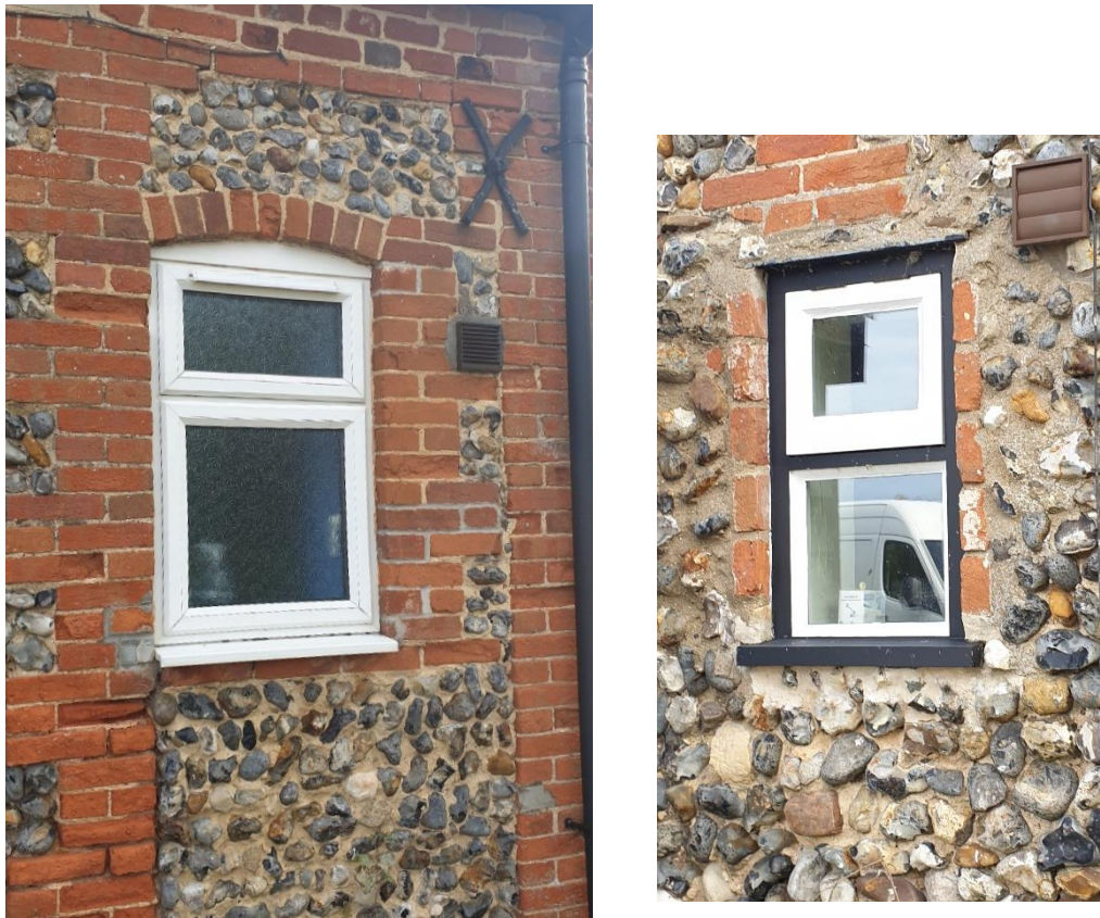
Figure 4: Existing uPVC window (left) and adjacent timber window (right)
