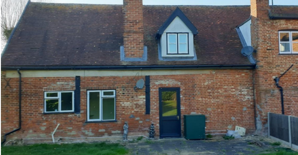
Figure 5: Existing door and windows to Eastern elevation
