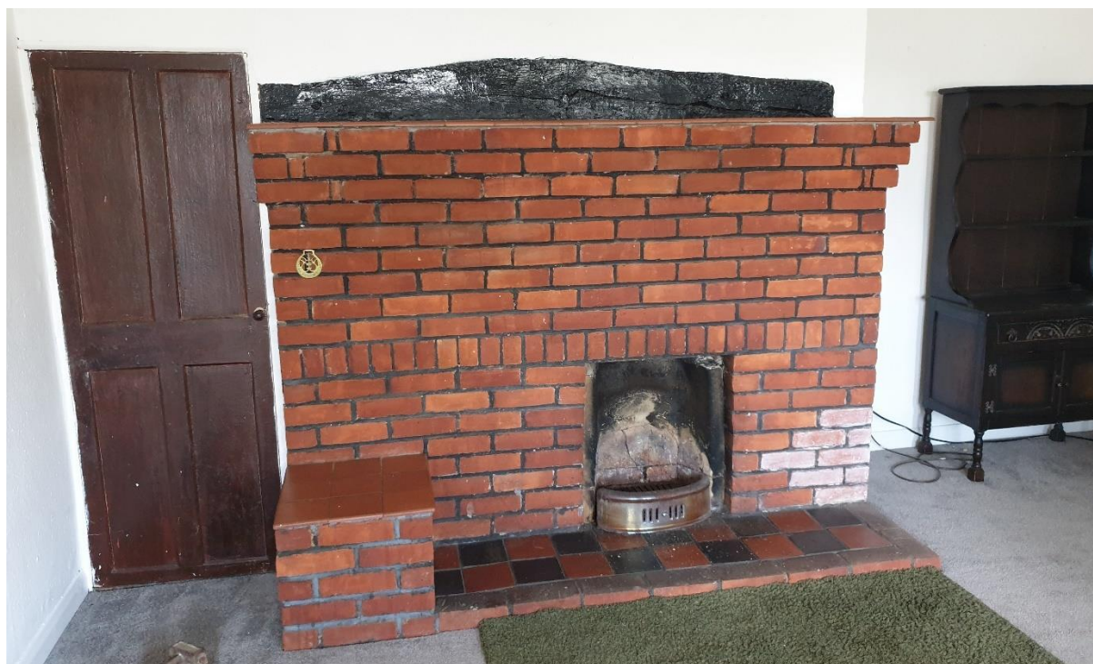
Figure 3: Altered Fireplace in Living Room
