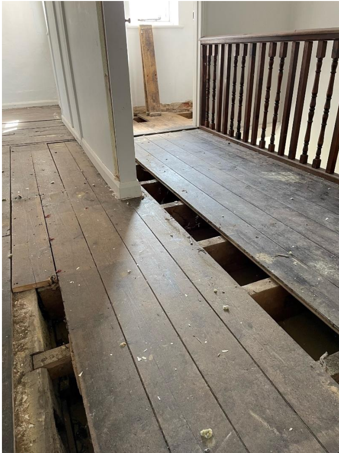
Figure 2b: Existing Landing & WC showing modern softwood joists
