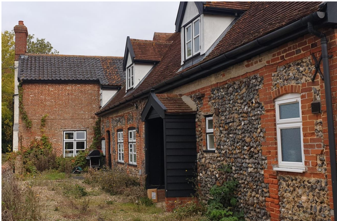
Figure 6: Existing Porch to Old Hall Cottage
