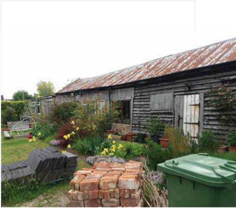
General Site Photo 3
