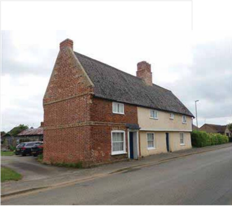
General Site Photo 1
