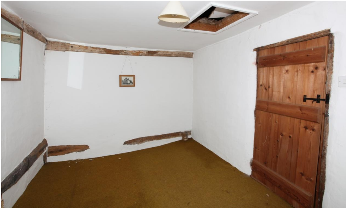
Illus. 23. The rear wall of the bedroom over the kitchen with the north-eastern gable to the left. A jowled post with an upstanding tenon for a missing tie-beam is visible in the right-hand corner, immediately opposite that shown in illustration 8. The roof-plate lies above the area of external weatherboarding in illustration 11 but is interrupted by a section of decay that would normally relate to a junction with another structure adjoining at right-angles. There is no evidence of any such structure on early maps.
