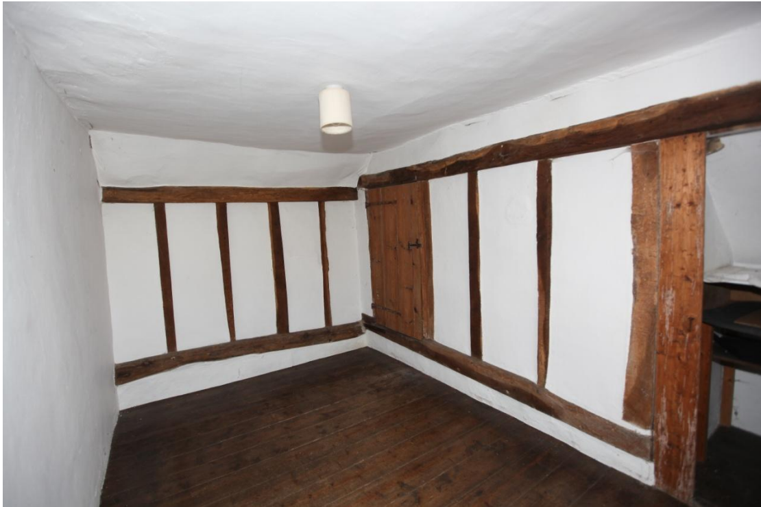
Illus. 25. The south-western bedroom (3) with no evidence of the single-storied roof in the gable on the right despite the presence of a lower tie-beam which also appears to have been renewed when the upper storey was added – as does the lower roof-plate of the back wall to the left. The good 19 th century pine doors open into cupboards in the brick lean-to alongside the chimney.
