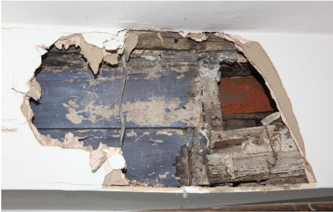
Illus. 11. A detail of the exposed external weatherboarding in the bathroom (illus. 10). The blue paint behind the modern plasterboard would have decorated the internal walls of the lean-to but the whitewash beneath may indicate the original external appearance of the building. The horizontal timber above is the original roof-plate visible internally (illus. 23) and the boarding respects the jamb and projecting lintel of a former door or window adjoining the corner to the right. This fragment suggests the entire house was weatherboarded initially and investigation above the lean-to ceiling may reveal whether it was confined to the lower storey.
