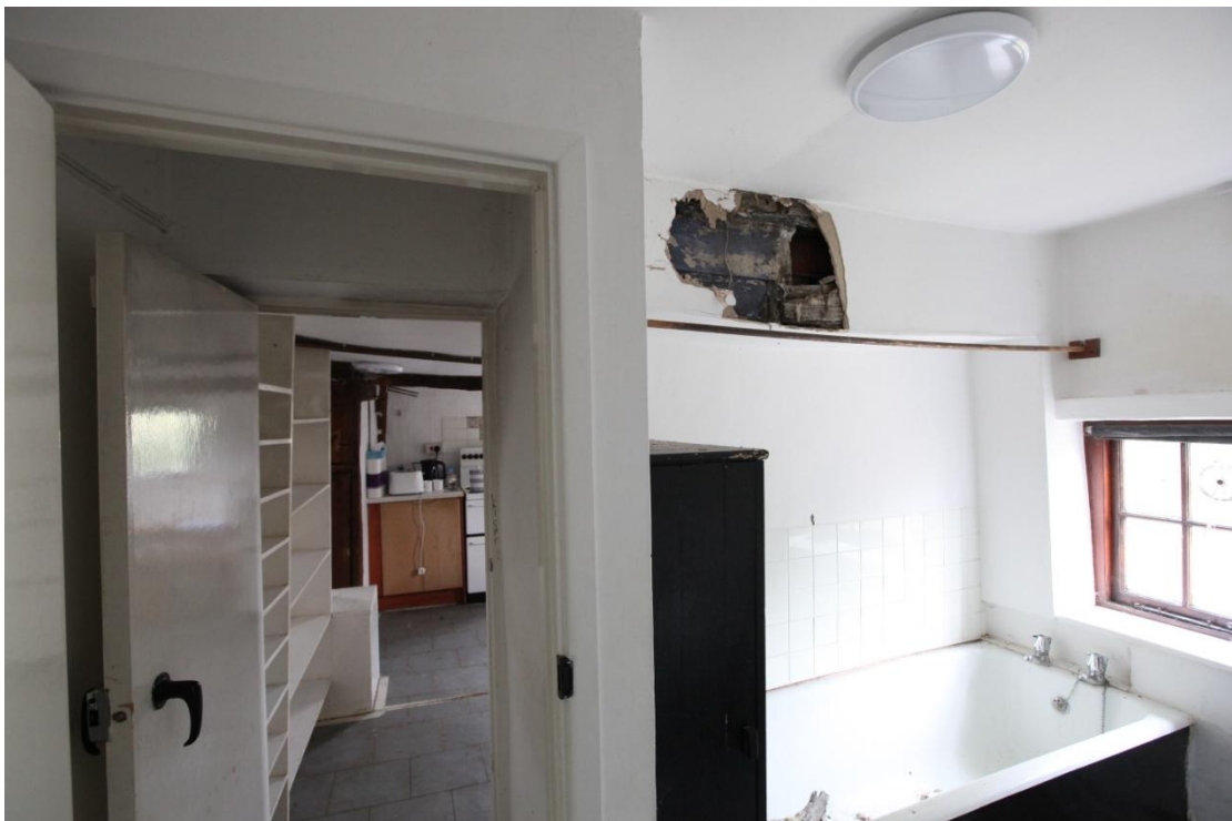
Illus. 10. The bathroom in the rear lean-to looking north-west towards the kitchen with part of the original weatherboarded external wall exposed on the right (see illustration 11). The lower section of this wall has been at least partly removed to create the recess that now accommodates the bath and the exact nature of what survives in the partition against the kitchen is unclear. It may represent only a late-20 th century replacement.
