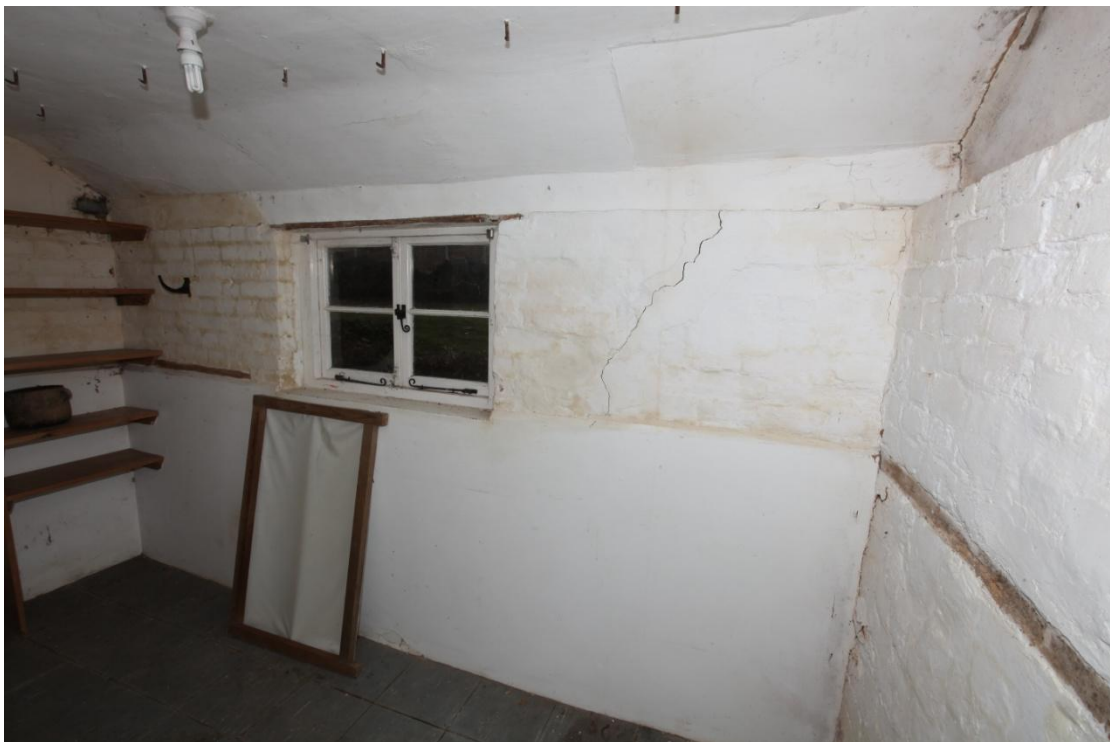
Illus. 20. The southern western internal wall of the gable lean-to which was shown for the first time on the Ordnance Survey of 1884. The 19 th century casement window is similar to that of the present bathroom and is one of the few that survived the late-20 th century refurbishment.
