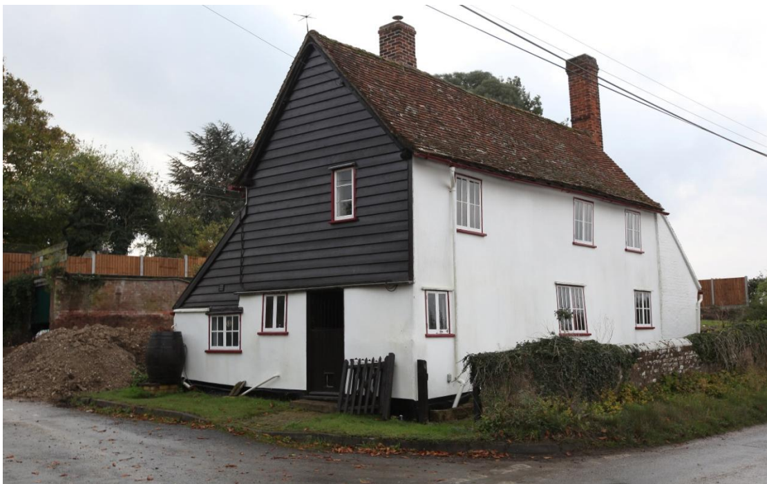
Illus. 2. The weatherboarding of the north-eastern gable facing Church Lane is a recent replacement of that shown in 1967 although the early-20 th century window to the first-floor bedroom survived the subsequent refurbishment along with that of the lean-to.
