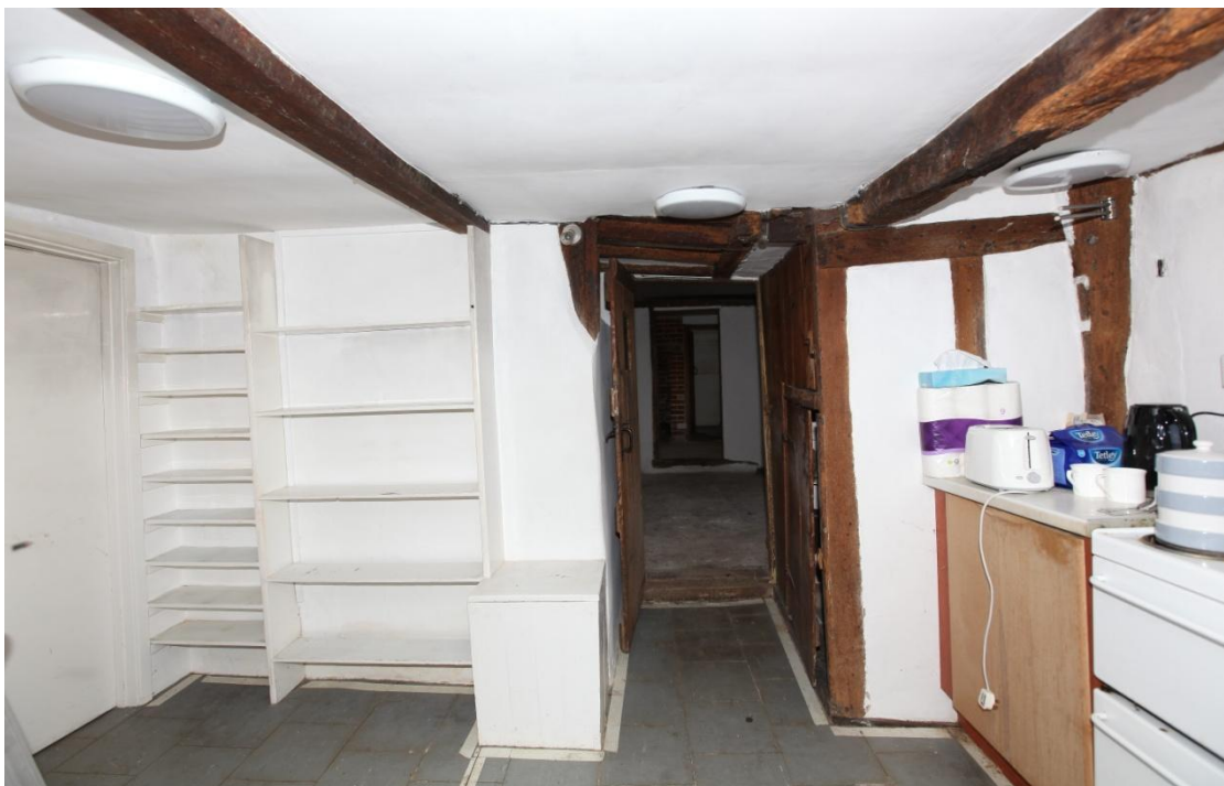
Illus. 6. The kitchen from the present entrance door in the north-eastern gable with the stair on the right and the 20 th century shelving attached to the back of the dining room fireplace on the left. The two axial joists differ in character and suggest the common joists have been altered or consist of re-used timber. Figure 9 shows the outline of a 19 th century cottage door in the front wall to the right.
