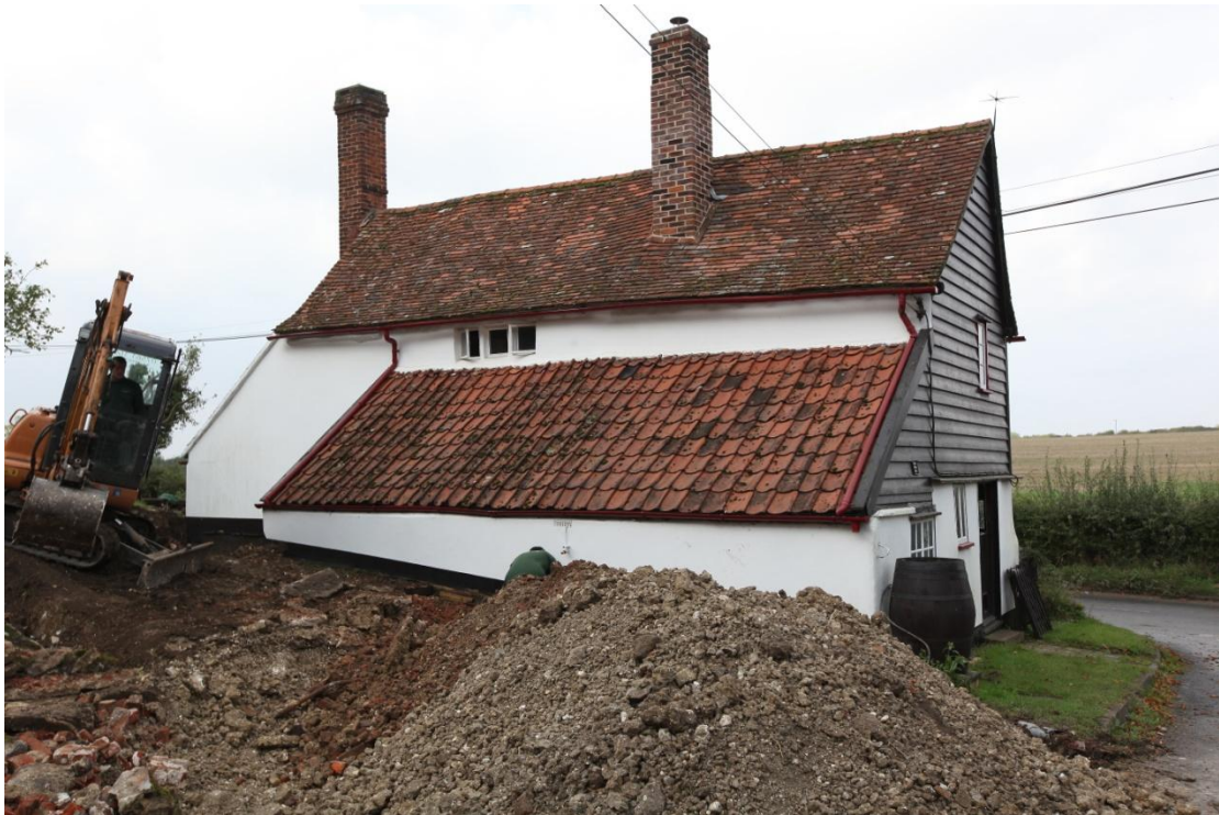
Illus. 4. If the Ordnance Surveys are accurate, the pantiled rear lean-to originally extended to the left-hand gable of the timber-framed building to leave only the brick lean-to projecting to the south-west. Although first shown on the Ordnance Survey of 1884 its walls are concealed by cement render and the extent of any subsequent rebuilding is unclear. It would be interesting to establish whether more of the earlier external weatherboarding is preserved within its roof than that shown in illus. 11.
