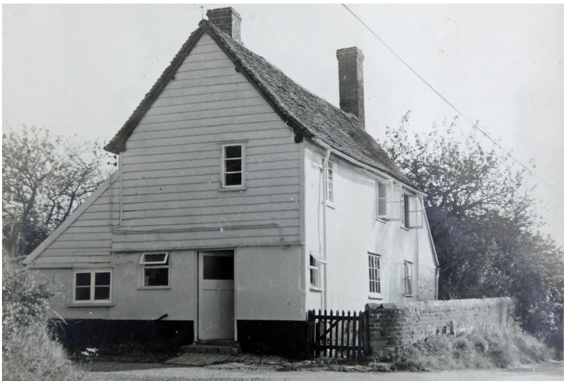
Figure 9. The property in 1967 from a photograph hanging in the house. A note to the reverse states that it was then owned and occupied by Pam and Bill Oldroyd. The gable door was probably a recent insertion as the dining room door had been blocked since 1961 and a new window cut into the front wall of the kitchen.
