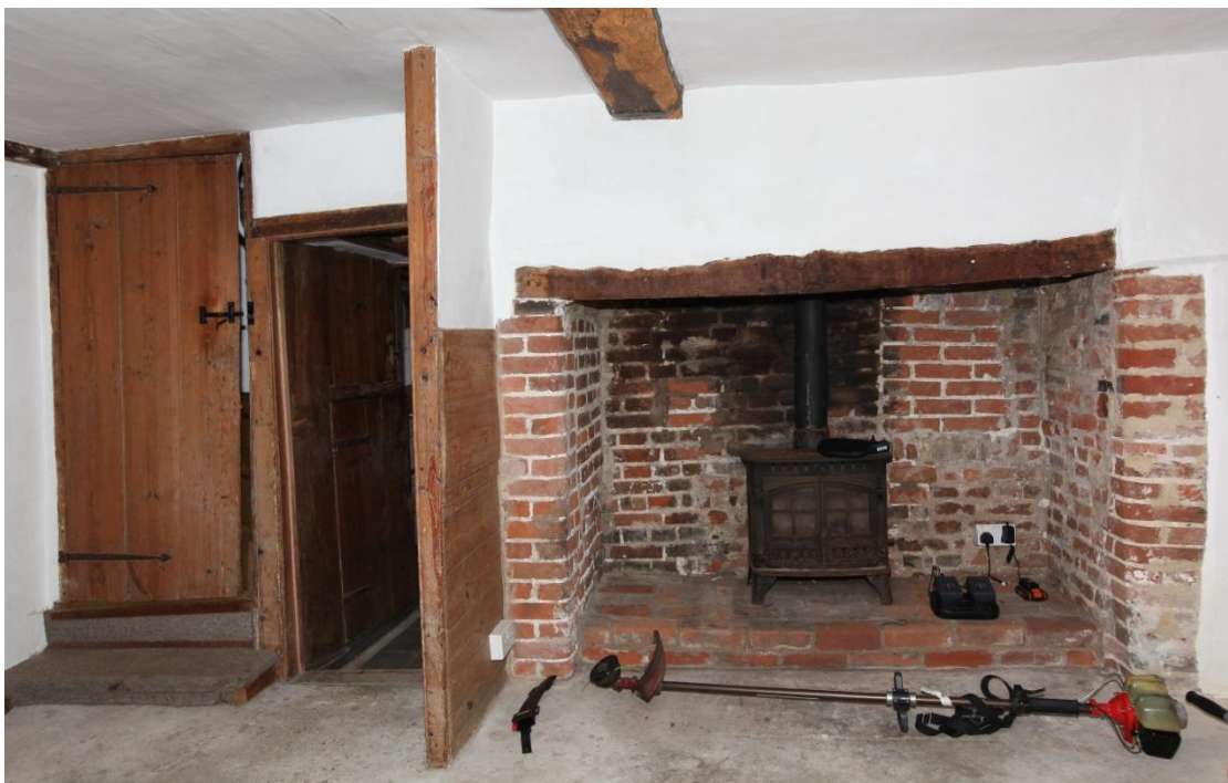
Illus. 14. The ‘dining room’ fireplace is impossible to date closely but is more typical of the 18 th century than either the late-17 th or early-19 th centuries. The pine boarding of the stair relates to the mid-19 th century remodelling as does the screen to the left of the fireplace which is intended to shield the occupants of the fireside from draughts and represents a rare survival.
