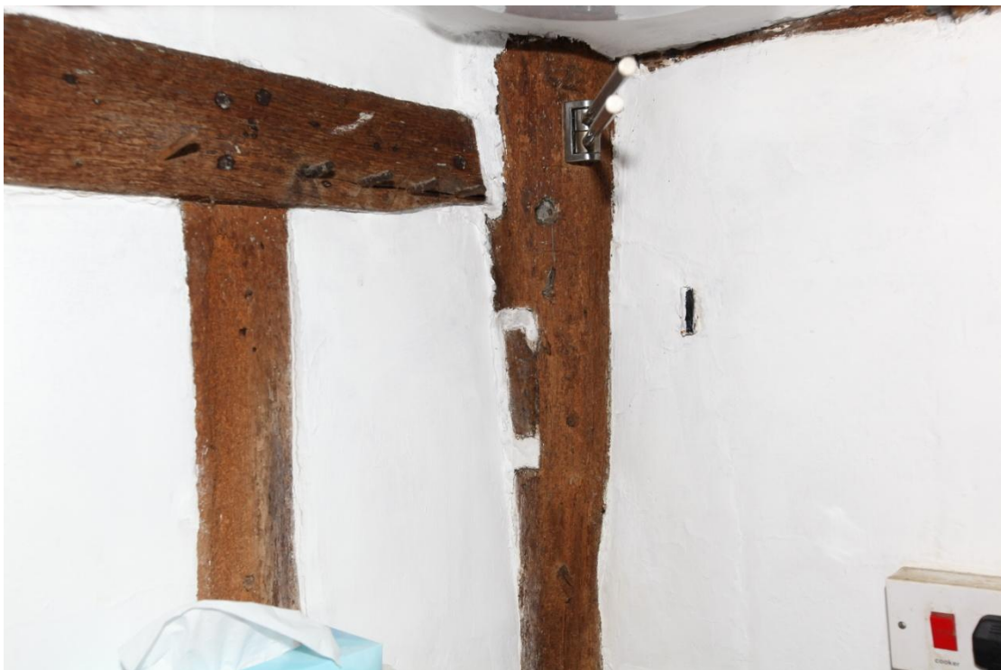
Illus. 8. A detail of the jowled storey post in the corner of the kitchen (illus. 7). This contains a pegged mortice for a missing lateral brace or mid-rail but is not respected by the present mid-rail which preserves a single pegged stud. These timbers all date from the 17 th century or before, but the extent to which the rest of the wall fabric is hidden by plaster makes it impossible to establish whether they remain in situ or have been re-used. The exposed timber at top-right is a rail supporting the ceiling joists.
