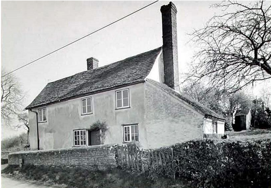
Figure 8. The house in 1961 with an entrance door in the front wall of the central ‘dining room’ as labelled in figure 10 and the outline of a blocked second door clearly visible in the right-hand corner of the present kitchen to the left (Royal Commission Archive). The windows have since been largely renewed with different glazing patterns.
