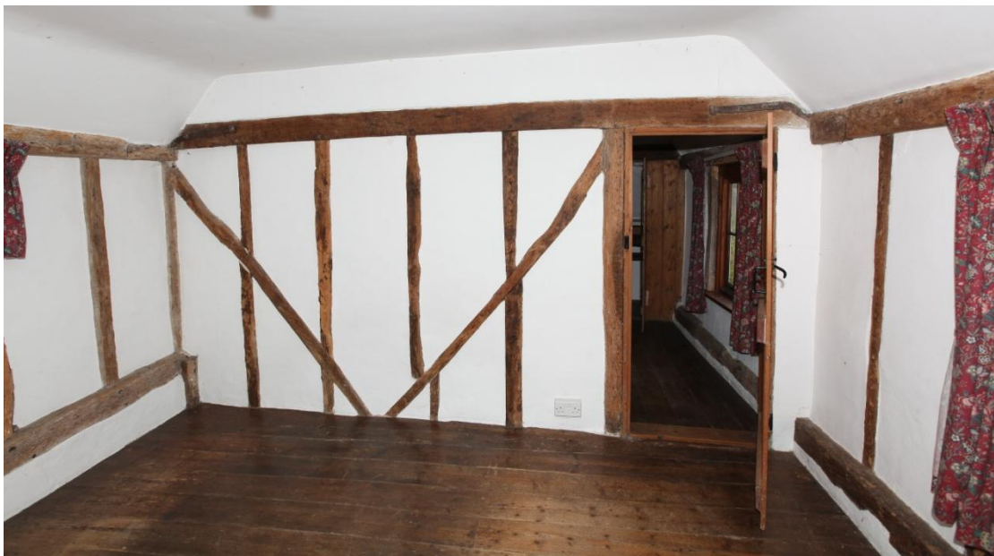
Illus. 24. The partition between the central bedroom (2) in the foreground and the south-western bedroom (3). Although the low roof-plates of the single-storied structure continue throughout, with a jowled post visible in the left-hand corner, the partition studs were replaced when the upper storey was added as there is no trace of the former roof. These studs are pegged to the upper tie-beam but their narrow proportions and straight diagonal primary braces respect the connecting door and are typical of the 18 th century. The front roof-plate on the right appears to be a 17 th century timber but its counterpart on the left contains pegs for studs above and beneath and was probably replaced when the upper storey was added.
