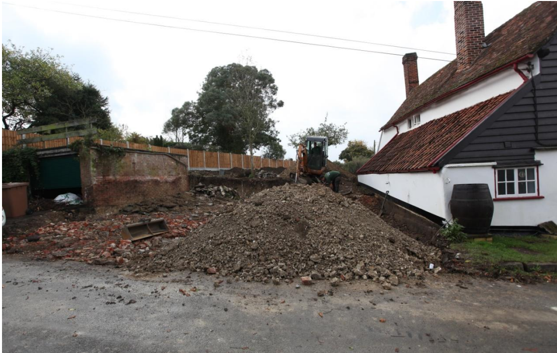
Illus. 3. The higher ground to the rear of the house reflects the slope of the hill into which the Fletton brick garage on the left was inserted at some point after 1970 (figure 7). The cement-rendered rear wall of the ostensibly brick lean-to on the right is straight rather than angled as depicted in figure 10.
