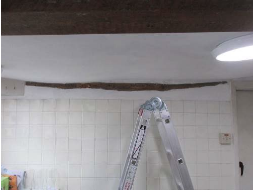
Photograph 17 – Modern fletton brickwork partition to be removed (100mm thick)
