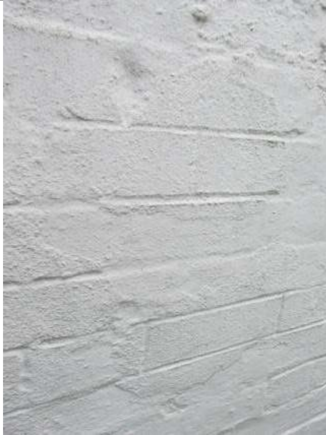
Photograph 09 – End lean-to cementitious render repairs to damaged brickwork, typical
