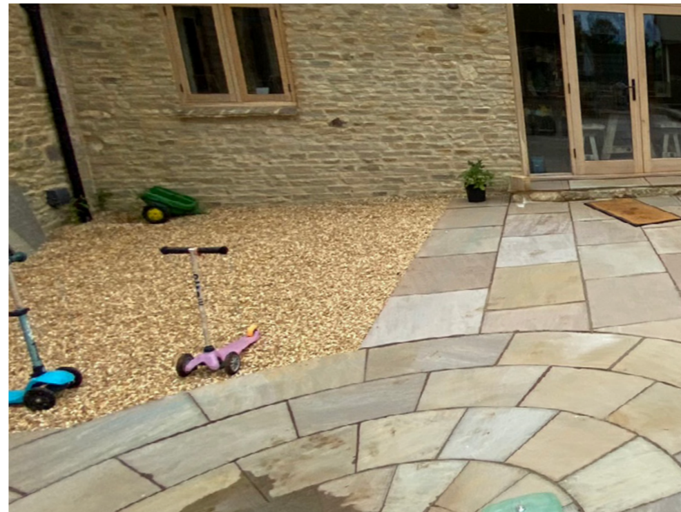
Patio areas - sandstone paving & pea shingle
