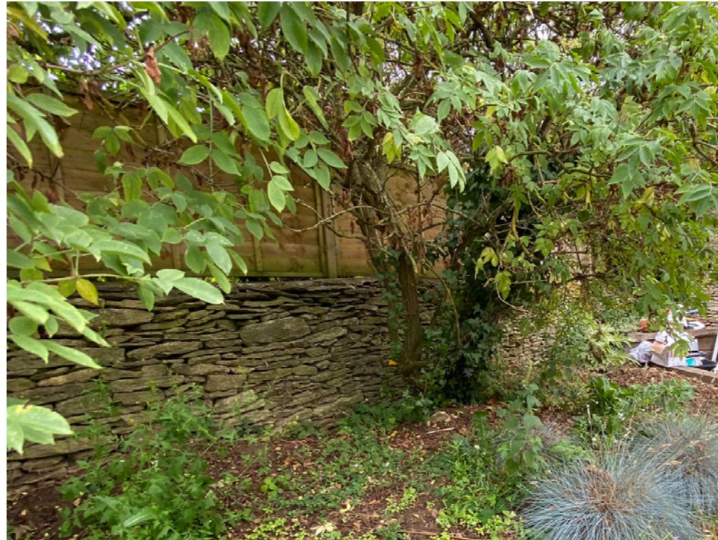
Original southern boundary 1.5m tall dry stone wall (section A)
