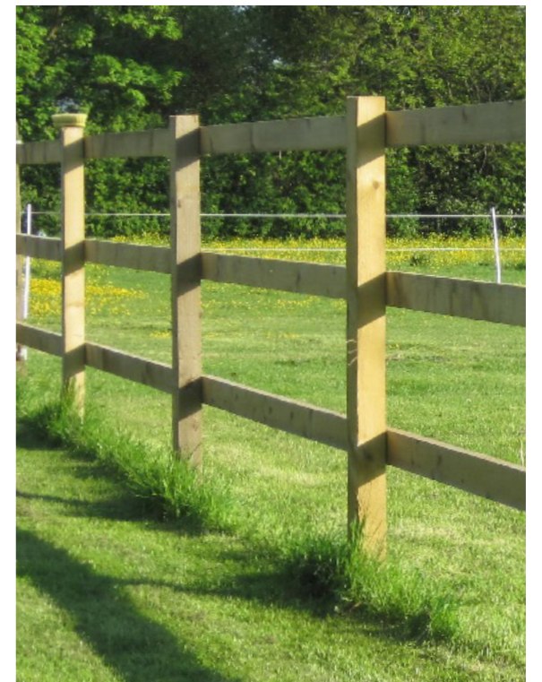
Example image of post & rail fence
