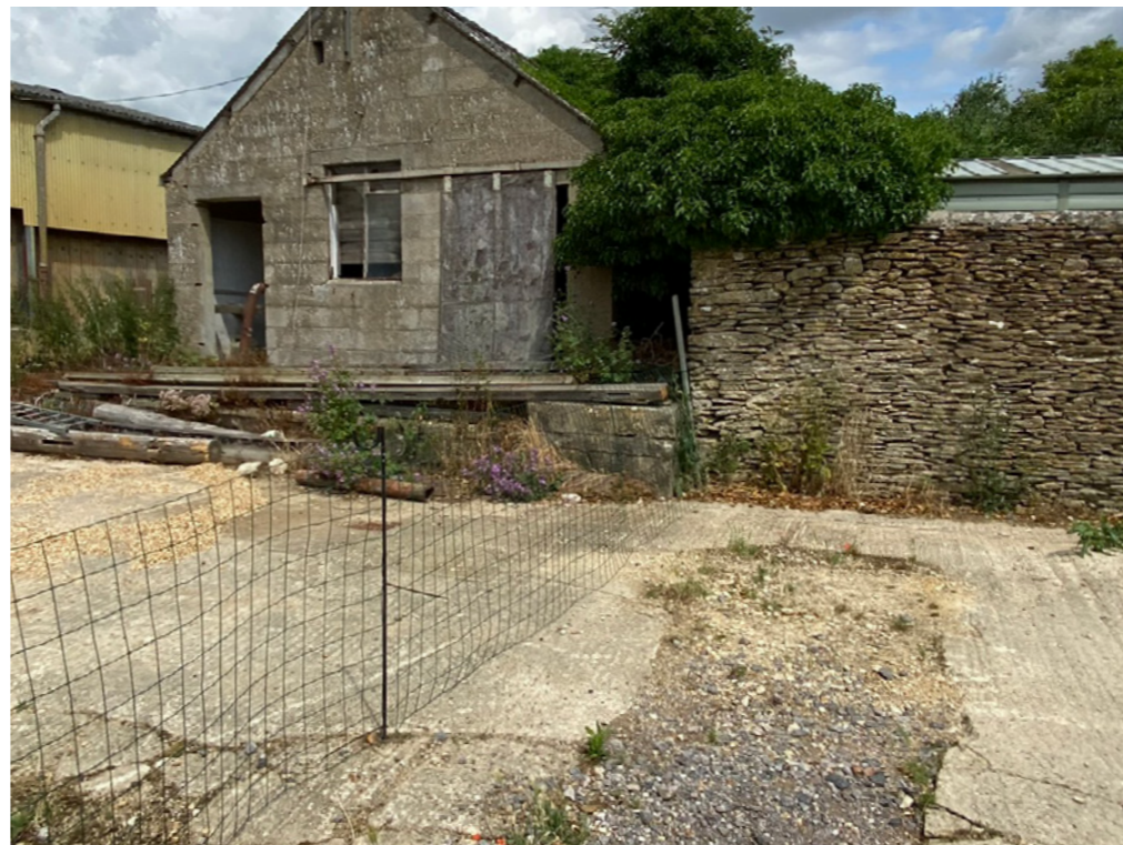
Entrance area original 2.3m tall dry stone wall & pig mesh fence. Pig mesh to be replaced with post & rail timber fence. Work to be completed in 2024
